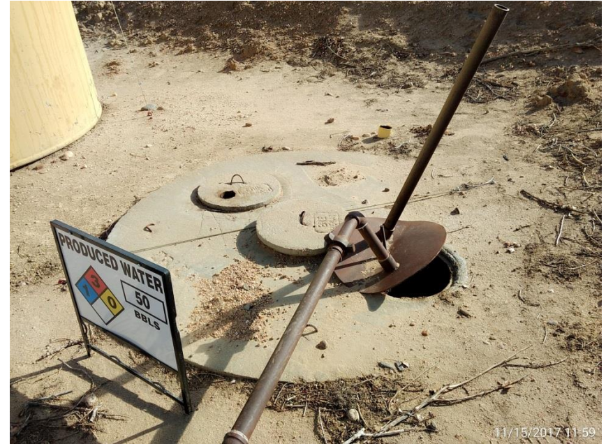
Produced Water Vault, Corrective Action: Water vault access bent open.
