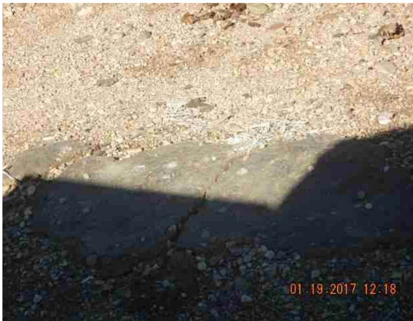
Photo from prior inspection for comparison
