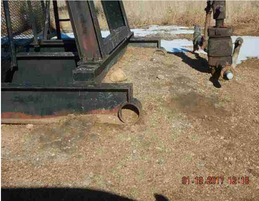
Photo from prior inspection for comparison
