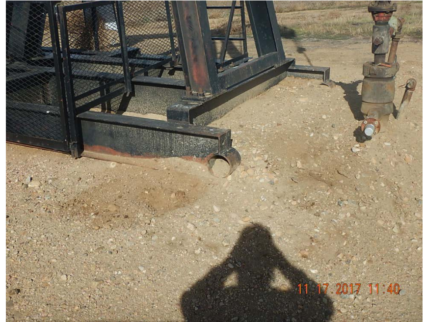
Photo 3: Stained soil removed
