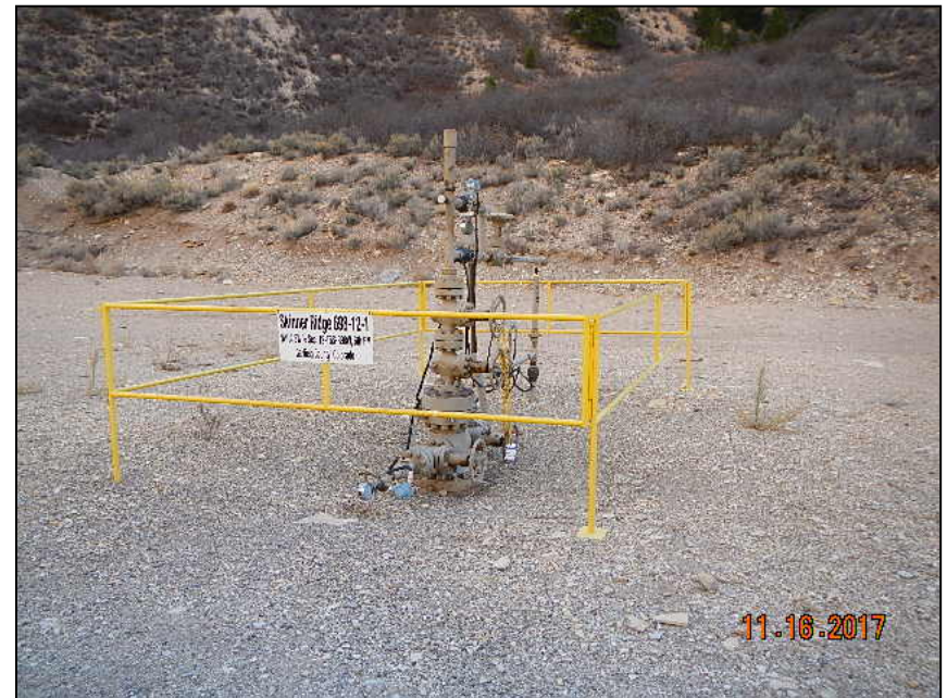
Photo 2. Wellhead. Hand wheels chained at time of inspection
