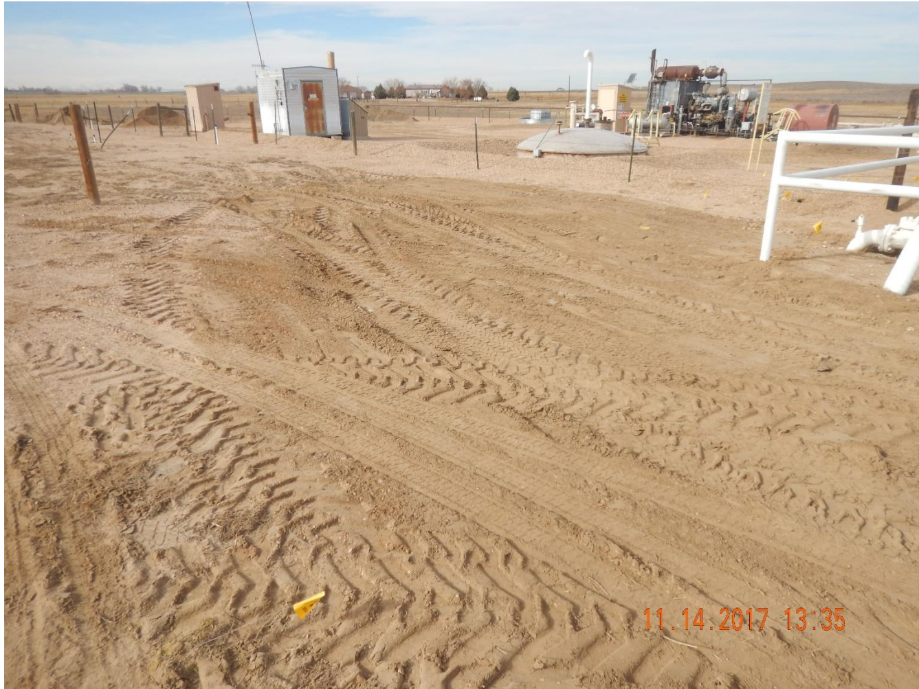
Photo 1: Photo taken from the east end of the former battery location. Photo shows all abandoned risers and equipment have been removed, and erosion has been repaired.
