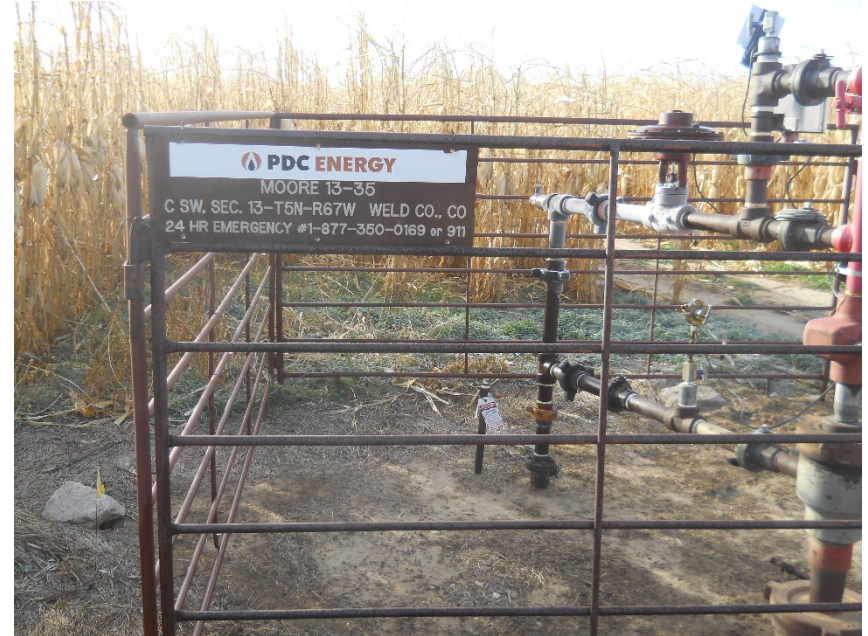
Wellhead looking south. 1" steel riser has been LOTO and labeled
