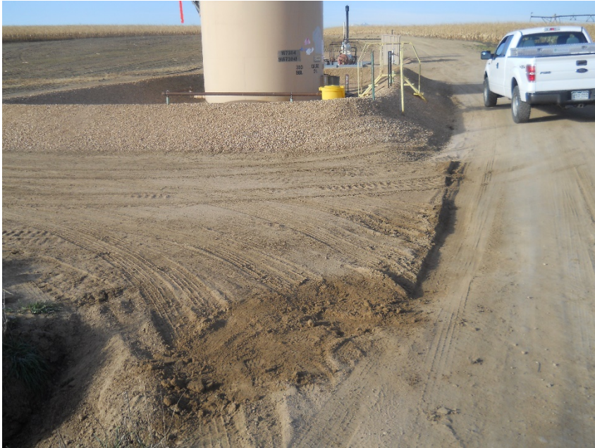
Northeast edge of location erosion has been repaired
