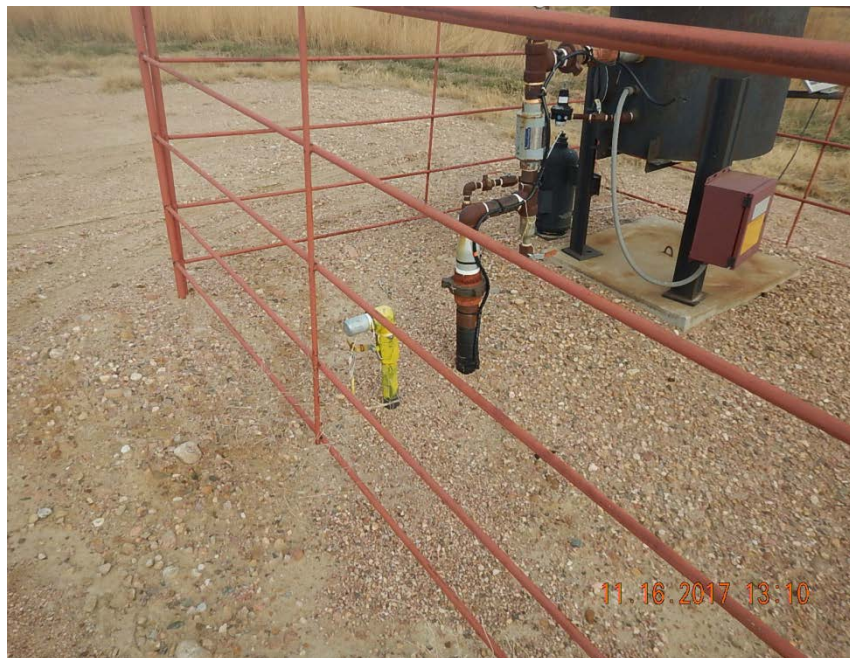
Photo 5: Marked riser, not in use at ECD
