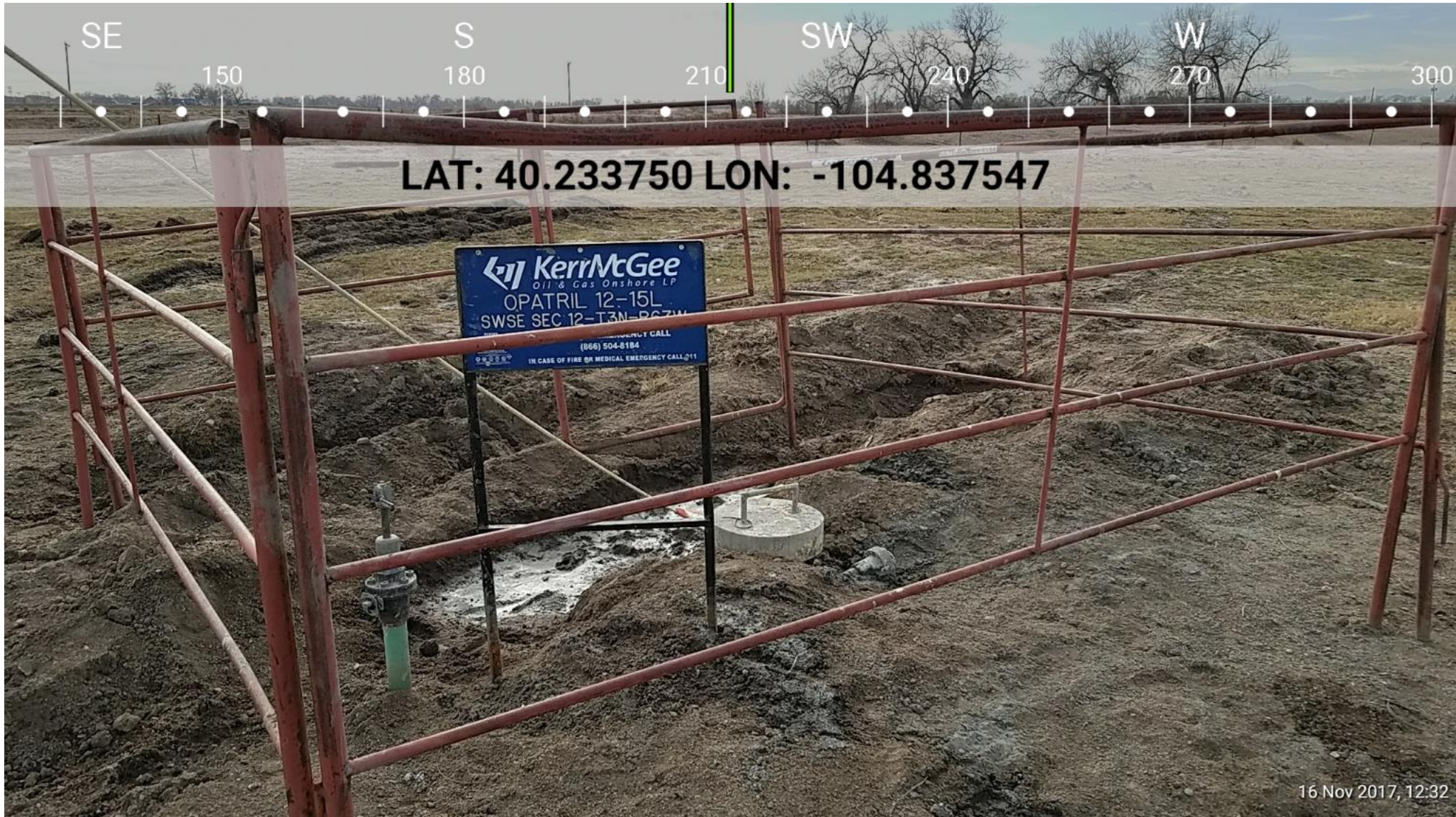
Wellhead API 05-123-15769 Location Number: 328259
