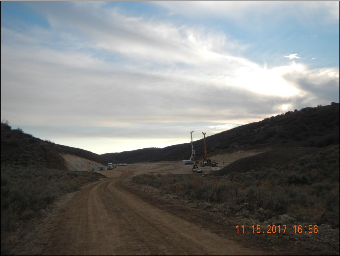
Location photo conductors being drilled.
