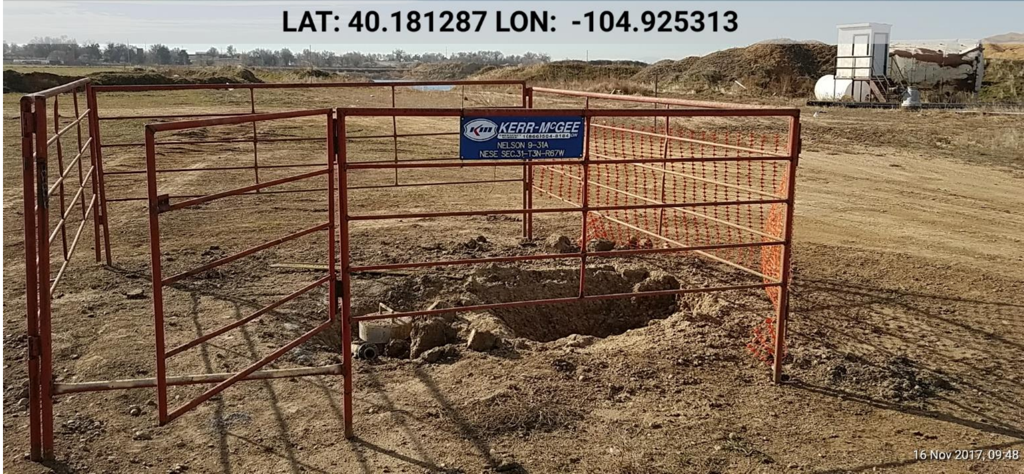
Wellhead (Plugged Awaiting Casing Cut) API 05-123-20670
