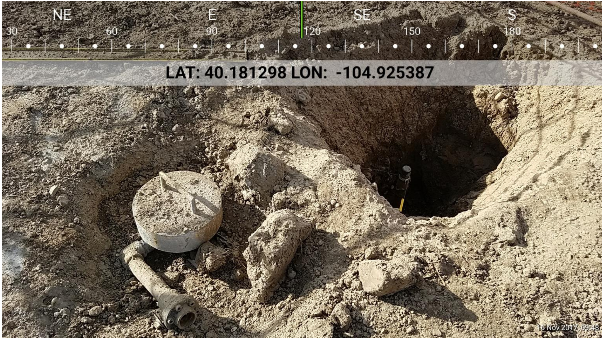
Exposed Wellhead and Flow Line
