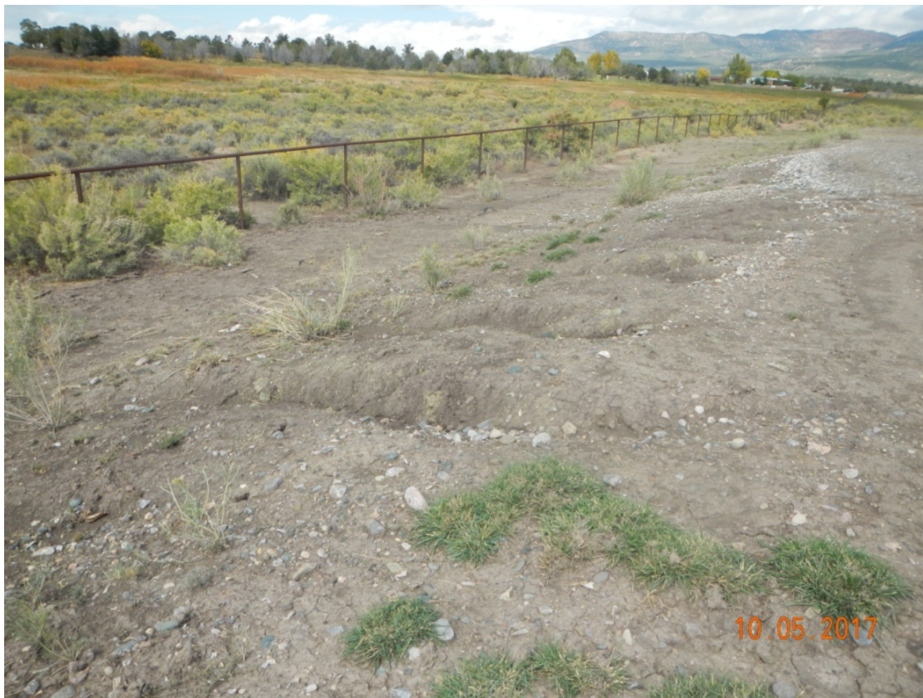
Photo 5. View of erosional channels in the southwestern portion of the project area.
