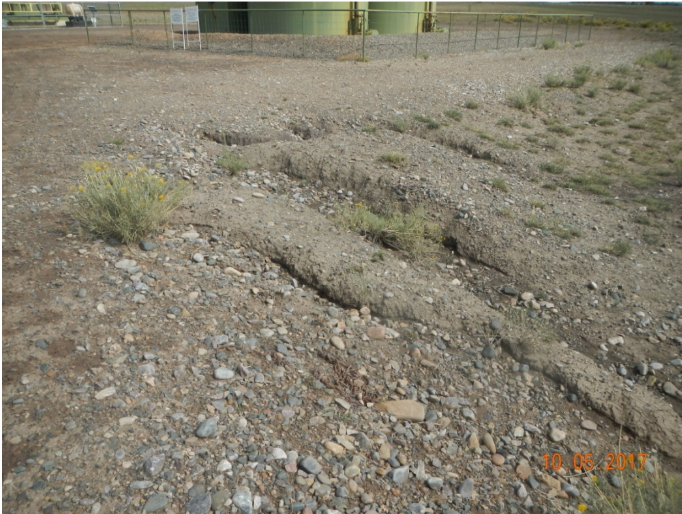
Photo 4. View of erosional channels forming near the well pad entrance. Stormwater controls need to be installed to stabilize erosion in eroding areas.
