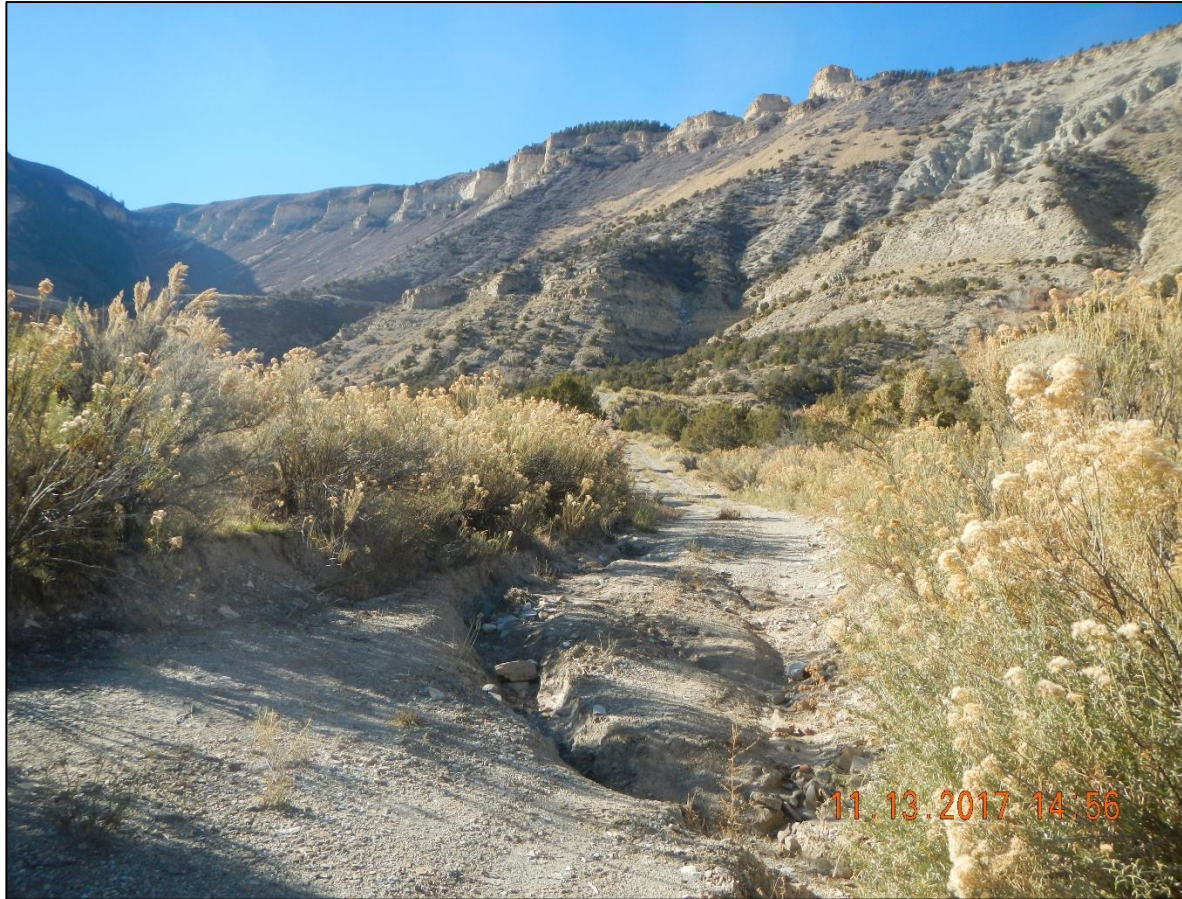
Deep erosion cut across access road.
