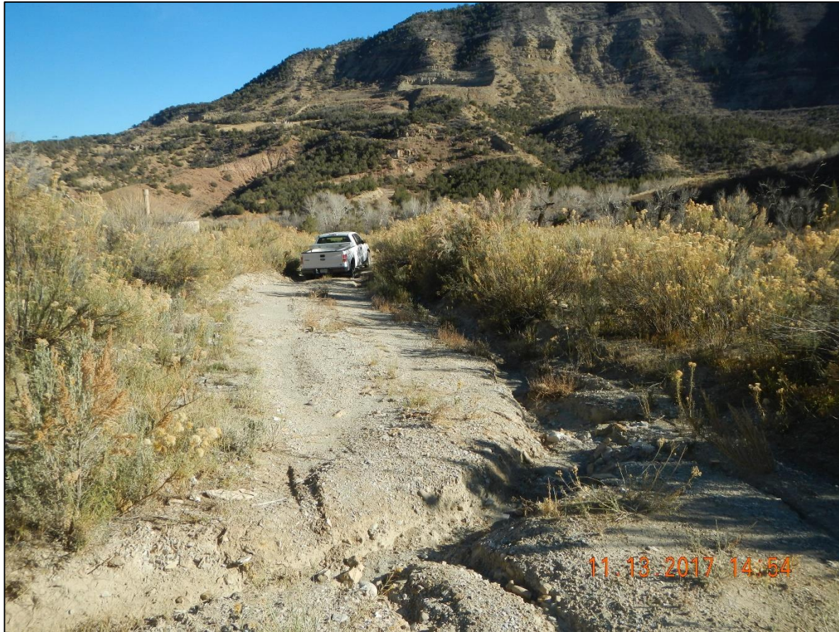
Deep erosion cut across access road.
