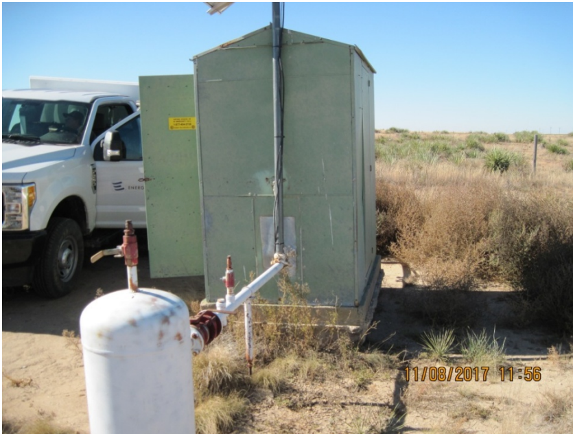
3. Meter shed and vertical gas separator
