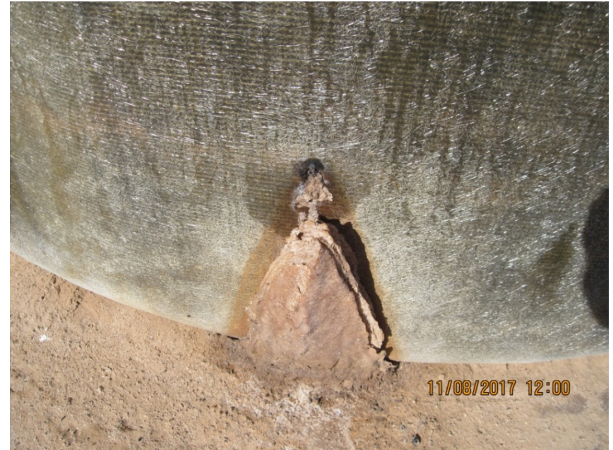
10. Water tank damaged and leaking
