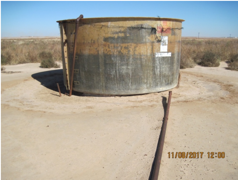
9. Open top water tank with no berms
