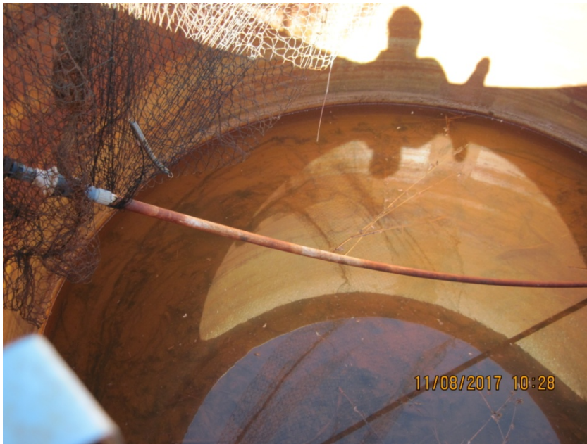
5. Inadequate wildlife netting, Fluid in tank 11/8/2017
