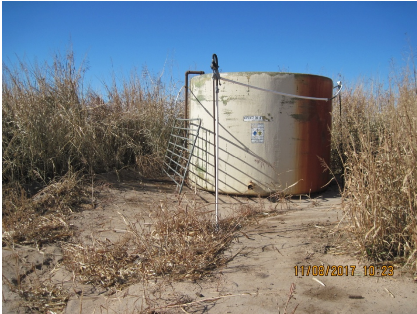
3. Water tank without berms 11/8/2017
