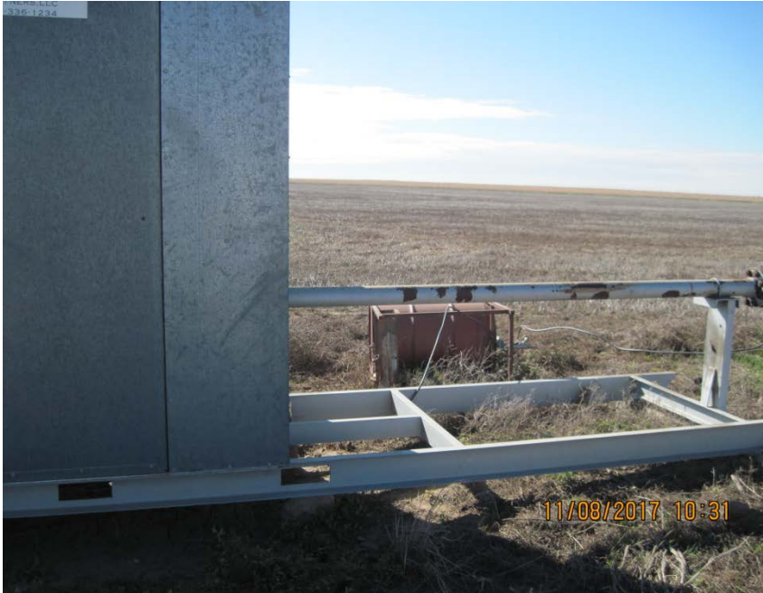
7. Chemical tank without containment (BMP) 11/8/2017
