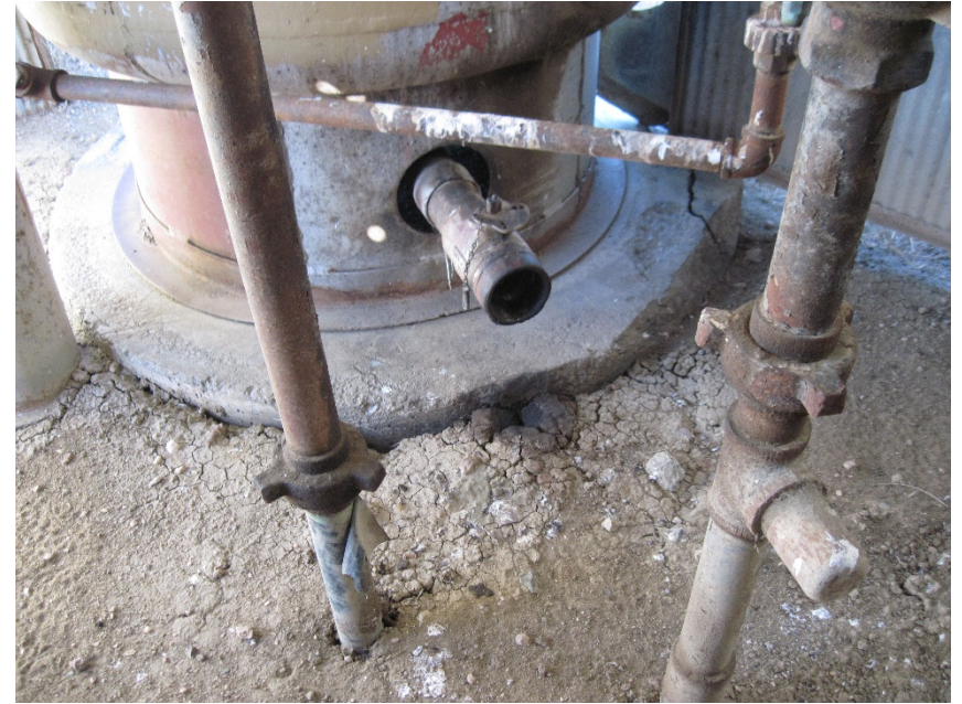
Valve leaking on treater
