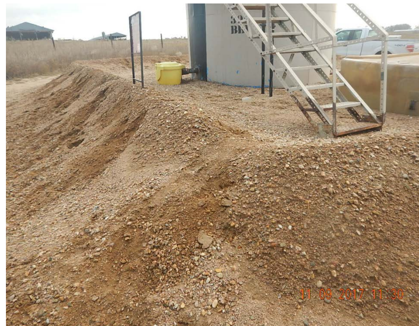
Photo 4: Low spot in berm
