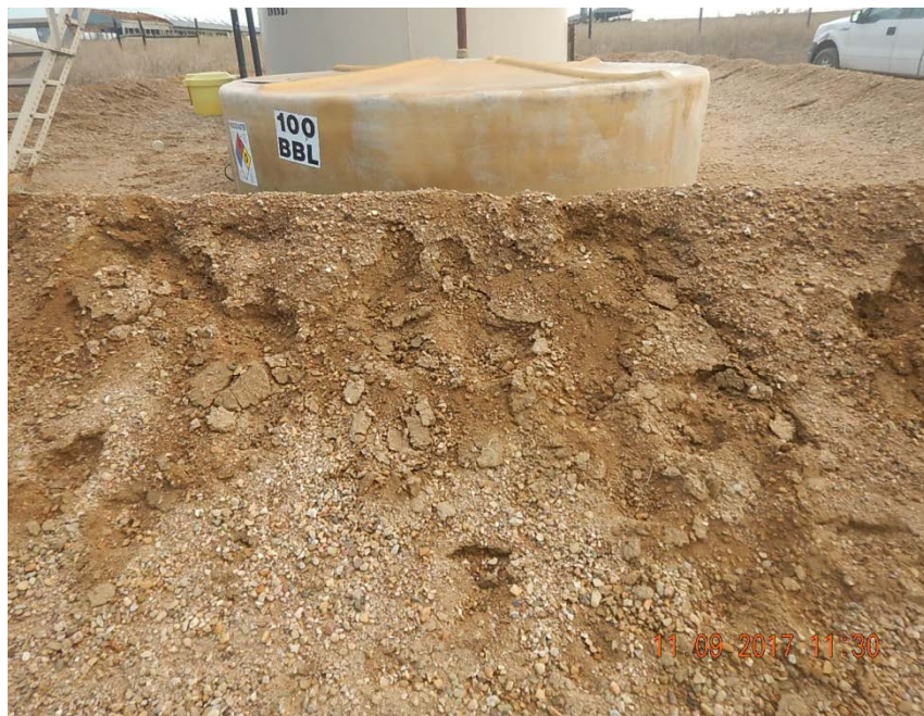
Photo 4: Damage on berm
