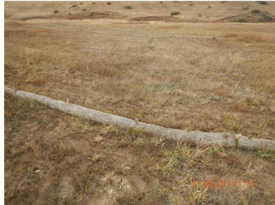
Photo 6: Photo taken from the south end of the location, facing southwest. Photo shows straw wattle ponding BMPs on location.
