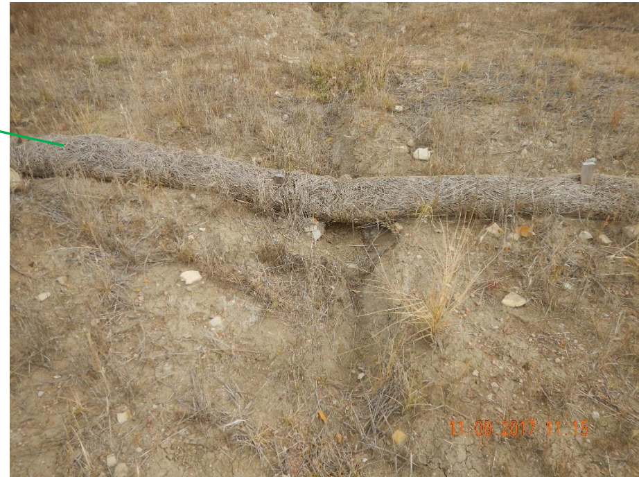
Photo 4: Photo taken from the straw wattle BMP at top of photo 3 (green arrow). Photo shows BMP is not longer in proper functioning condition as stormwater has cut under the wattle.
