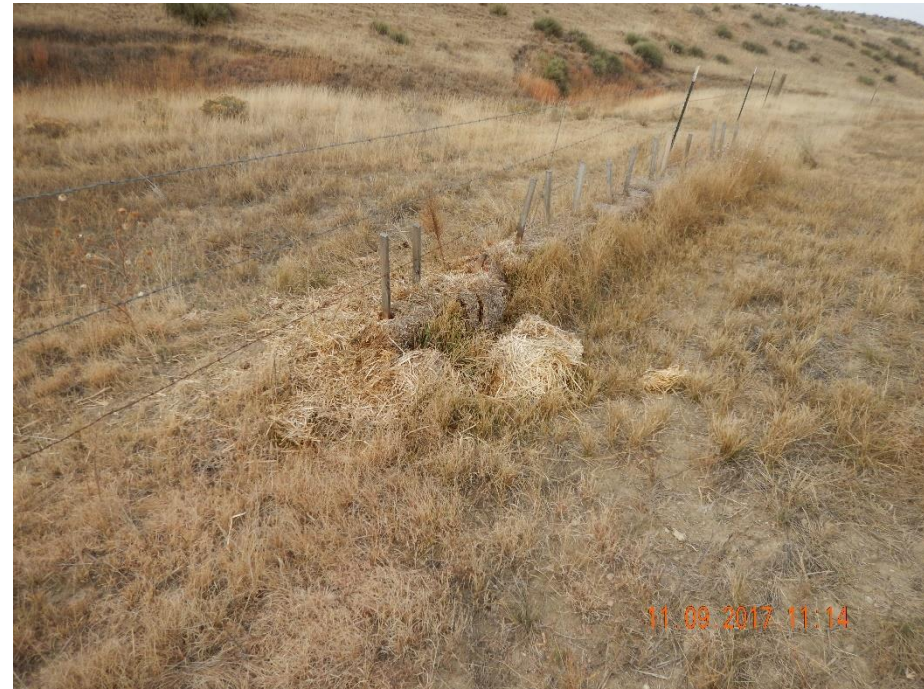
Photo 2: Photo taken from the southwest end of the location, facing west. Inspection #682502556 required operator to install or repair stormwater and sediment control BMPs on location. Photo shows hay-bale ponding BMP that has not been maintained or repaired, and is not in proper functioning condition.
