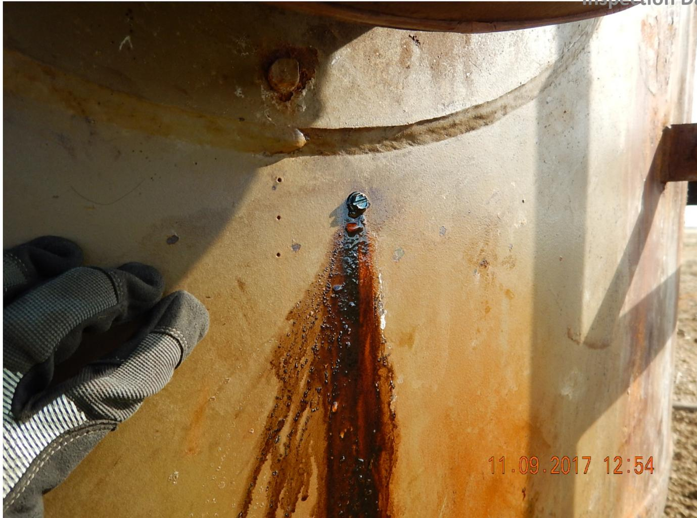
Attempted repair of hole in treater. Hole in treater is still leaking
