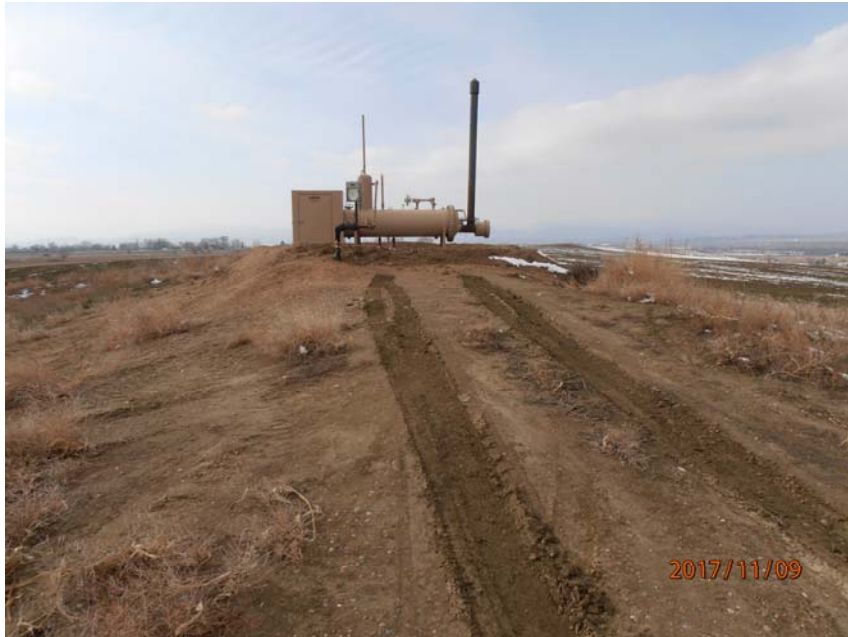
Photo 3: Horizontal Separator
