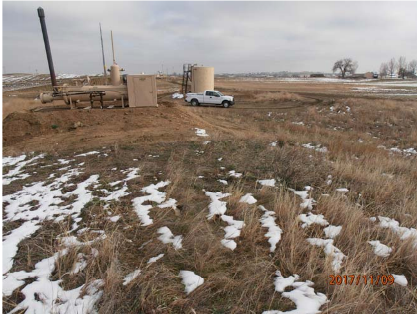
Photo 5: Tank Battery Viewing East
