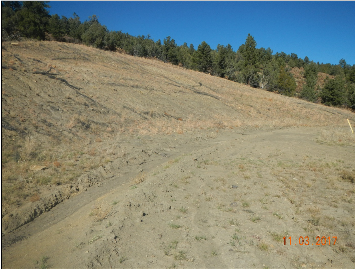
Photo 5. Facing north toward the cut slope. There is a ditch which has filled in with sediment at the base of the cut slope. The ditch divert stormwater toward the access road and southwest side of the location. No other BMP's are installed.
