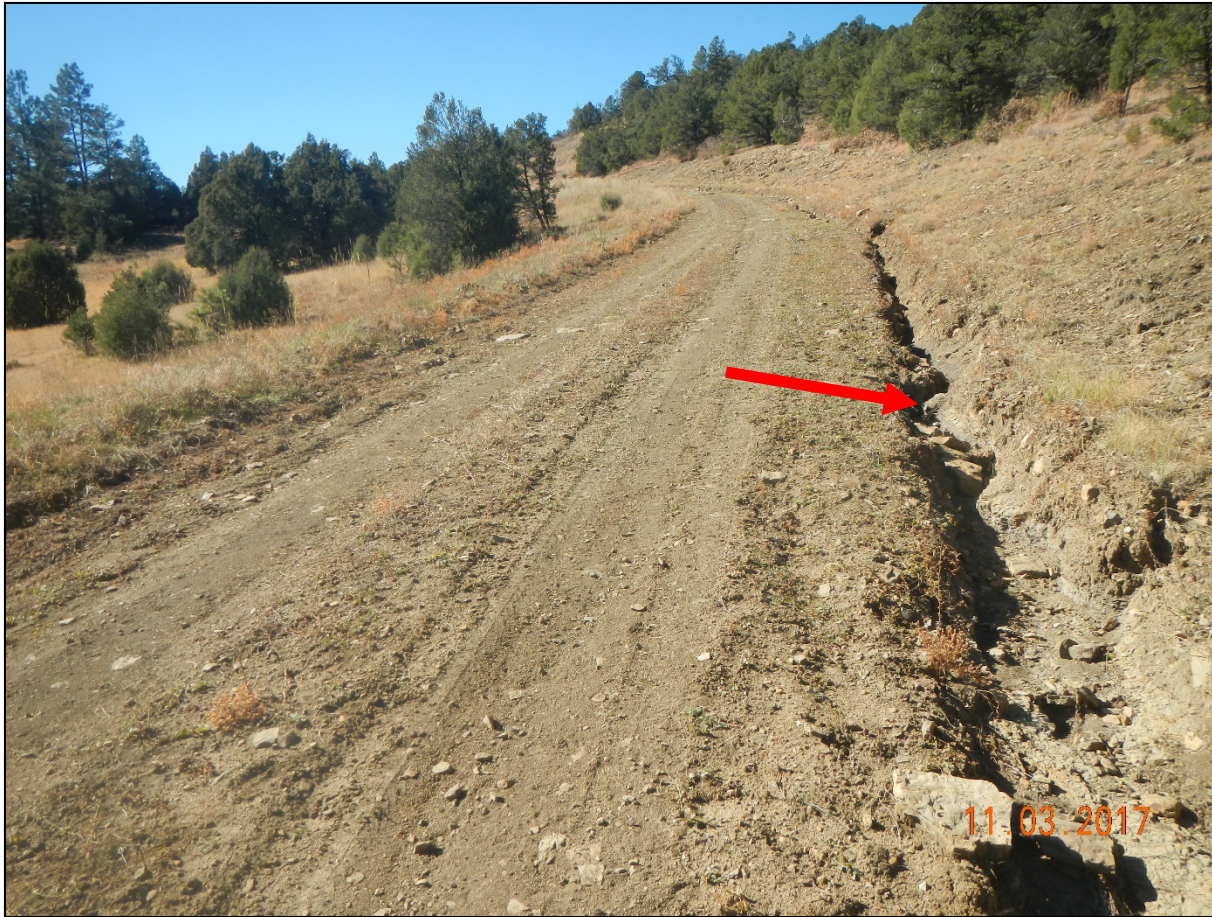
Photo 2. There are no BMP's installed along the access road. Stormwater erosion has incised the side of the road.
