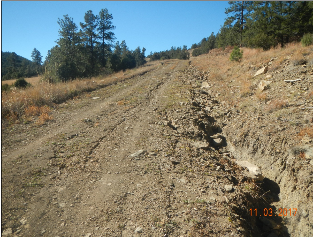
Photo 1. Facing southwest along the access road. There is stormwater erosion occurring down the access road. No BMP's are installed to prevent erosion.
