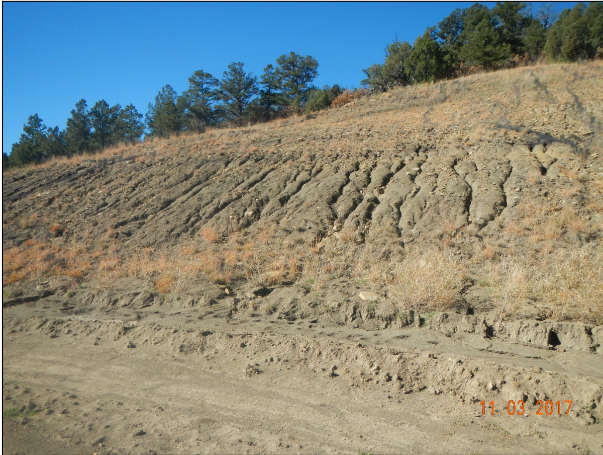
Photo 4. Facing toward the northwest cut slope which is not stabilized. Stormwater erosion is occurring along the cut slope.
