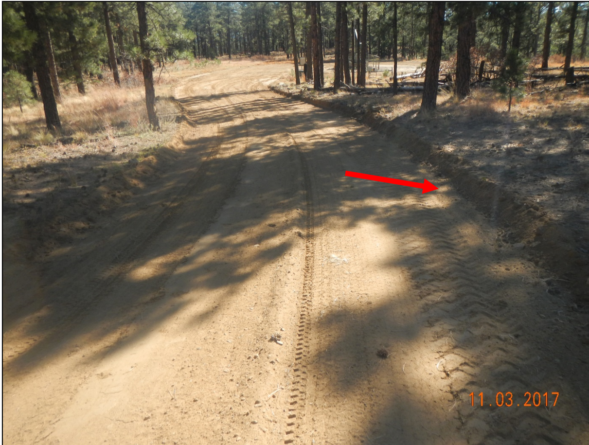
Photo 3. The arrow points to the side of the road cut where soil was pushed onto the road which is also causing the road to become widened. The grade of the road is being lowered by grading activities.
