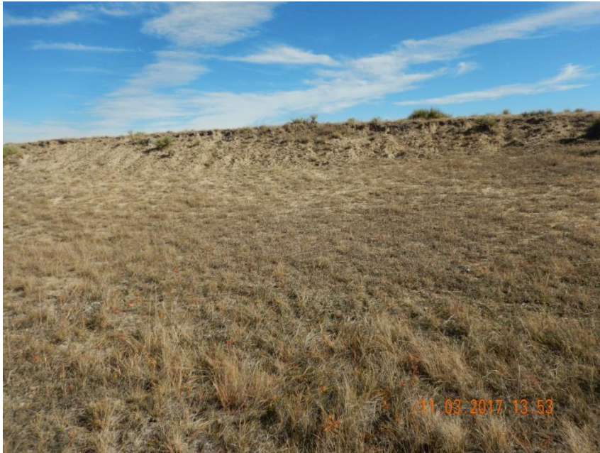
Photo 3. Photo taken of the eastern well location, facing East. Operator has not reclaimed the location per Rule 1004 standards. The location has not been contoured to match the surrounding landscape. Rill erosion evident along the eastern cut slope.
