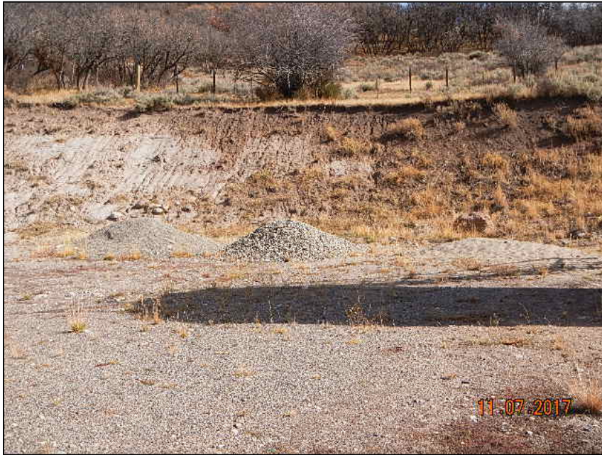
Photo 3. Stored gravel. Cut slope erosion.
