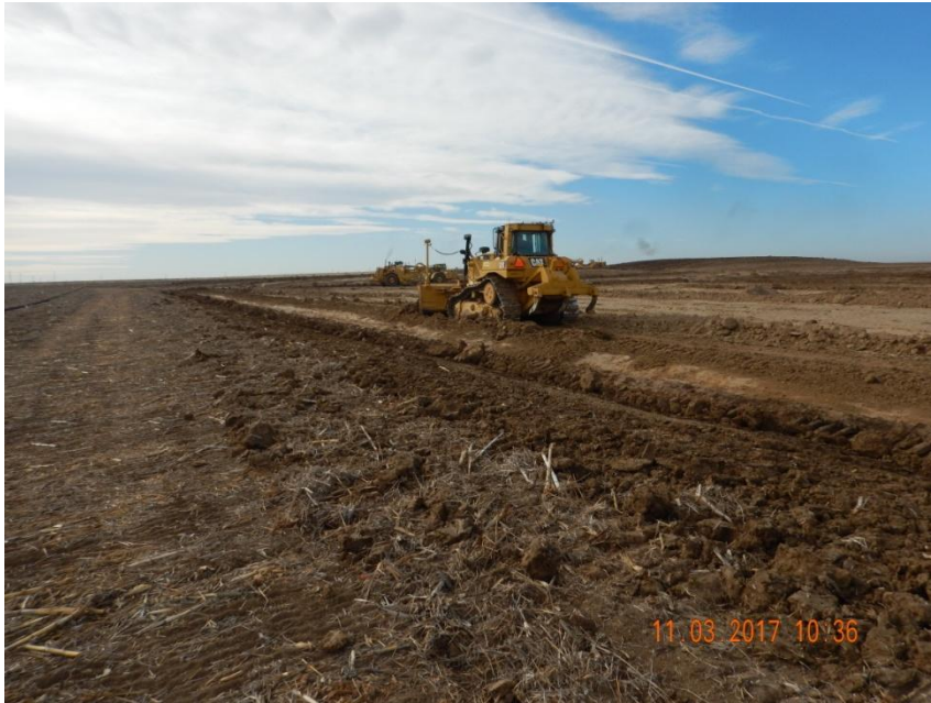
Photo 5. Photo taken from the eastern location, facing South. Topsoil salvage operations are IN-PROCESS.
