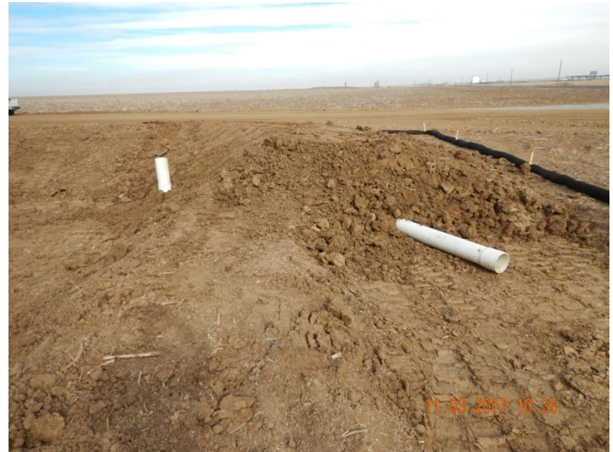
Photo 2. Photo taken from the northeastern location, facing North. Sediment trap is IN-PROCESS of being constructed. A temporary filter wattle BMP has been installed around the perimeter of the location.
