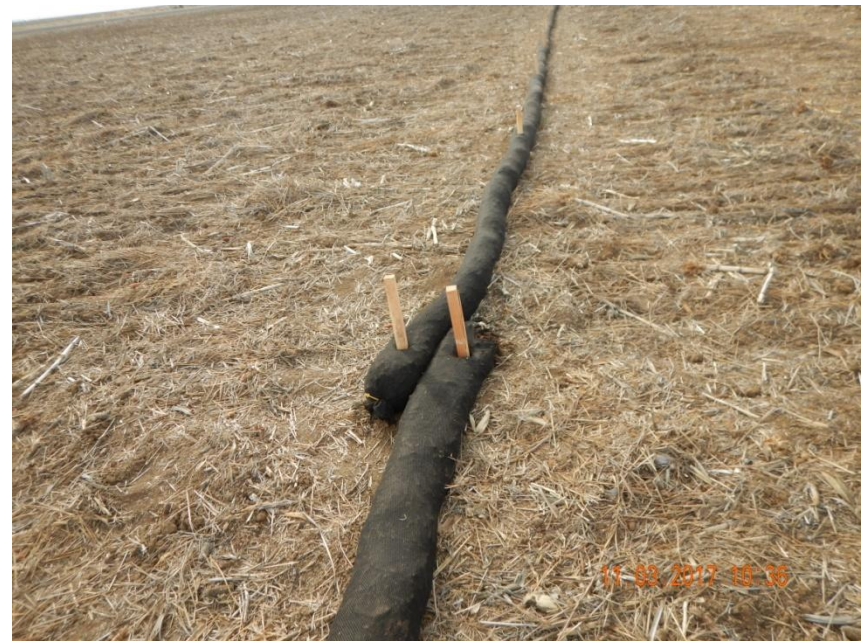
Photo 4. Photo taken from the eastern location. Photo illustrates the wattle BMP has been overlapped at the joints and properly staked.
