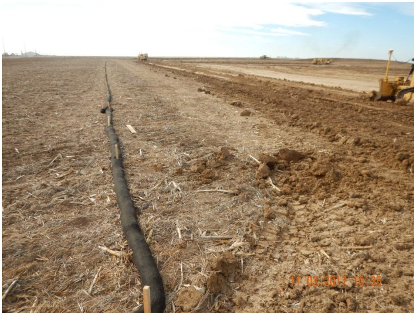
Photo 3. Photo taken from the northeastern location, facing South. Operator has installed a temporary filter wattle BMP has been installed around the perimeter of the location.
