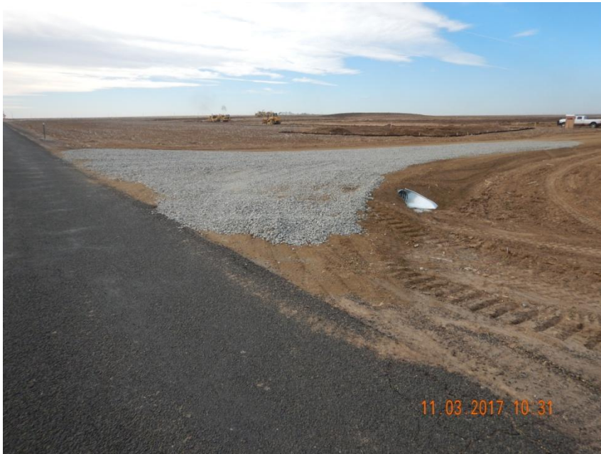
Photo 1. Photo taken from the entrance of location, facing South. Tracking pad device has been installed.
