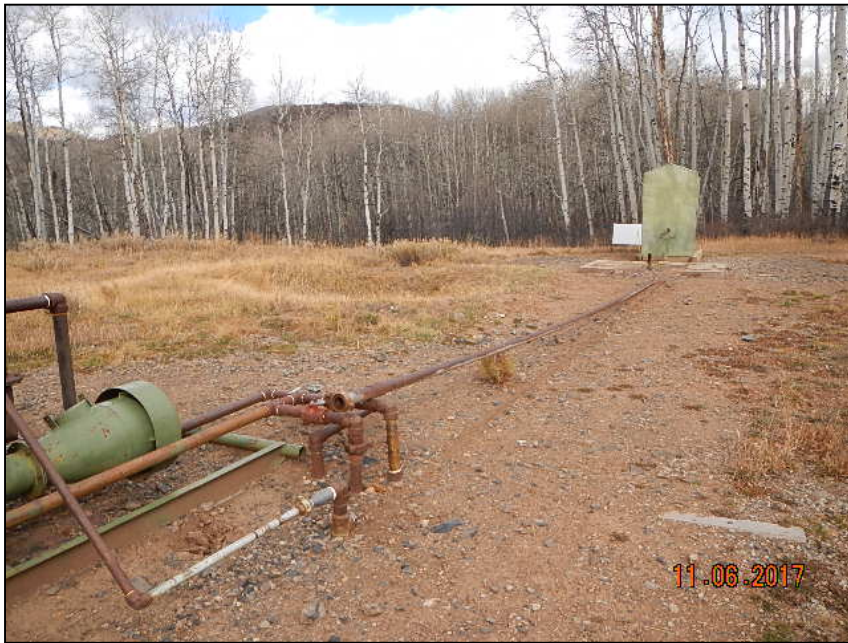
Photo 3. Disconnected line from separator to meter.
