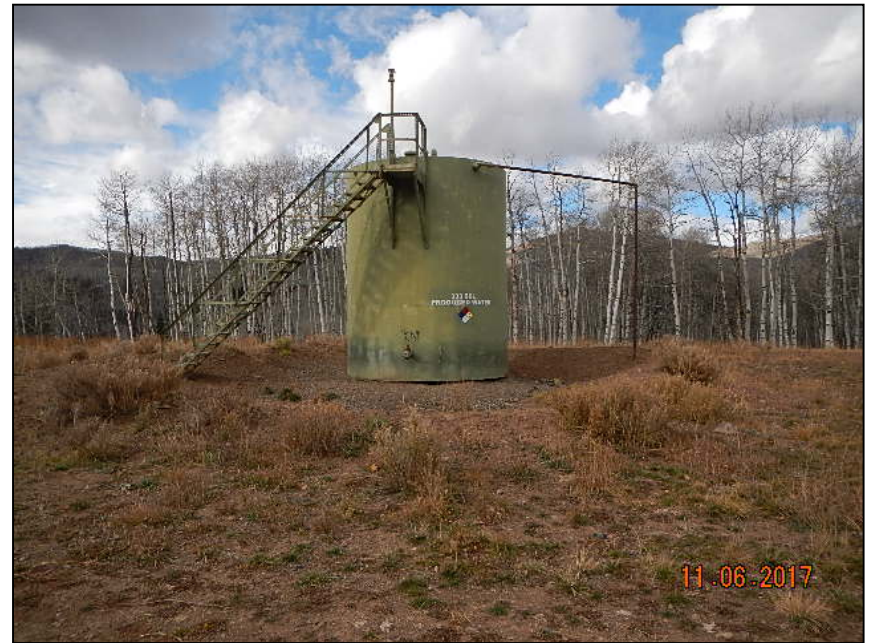
Photo 2. Vegetation and vegetation debris on berm and in containment.
