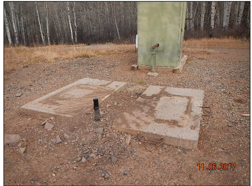
Photo 4. Unmarked riser and disconnected meter.
