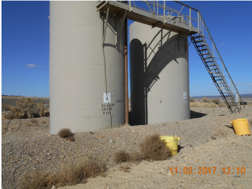
Produced water tanks
