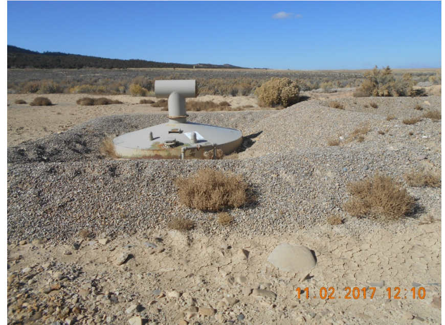
Partially buried condensate tank
