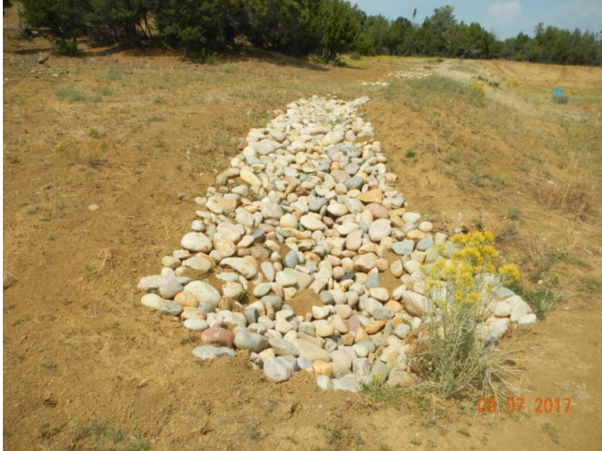
Photo 1: View of cobble stormwater controls installed in the western portion of the project area.
