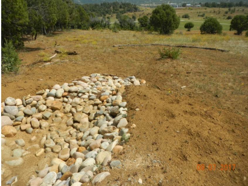
Photo 5: View of stormwater controls in the northeastern portion of the project area where stormwater flows eastward (toward the upper right-hand corner of the photo).
