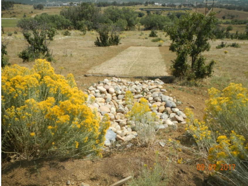
Photo 3: View of stormwater controls and erosion repair downstream from culvert outlet near the entrance of the well pad.
