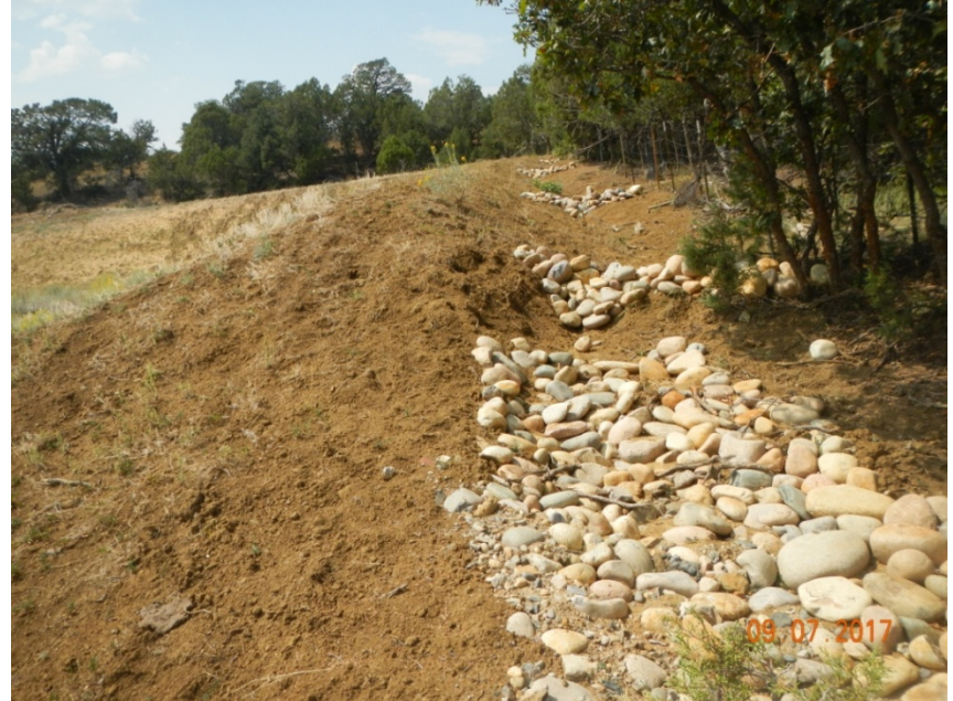
Photo 6: View of cobble stormwater controls in the northern portion of the project area, upstream of Photo 5.
