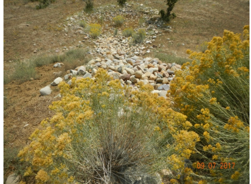
Photo 4: View of cobble run down and silt trap in the southeastern corner of the project area.
