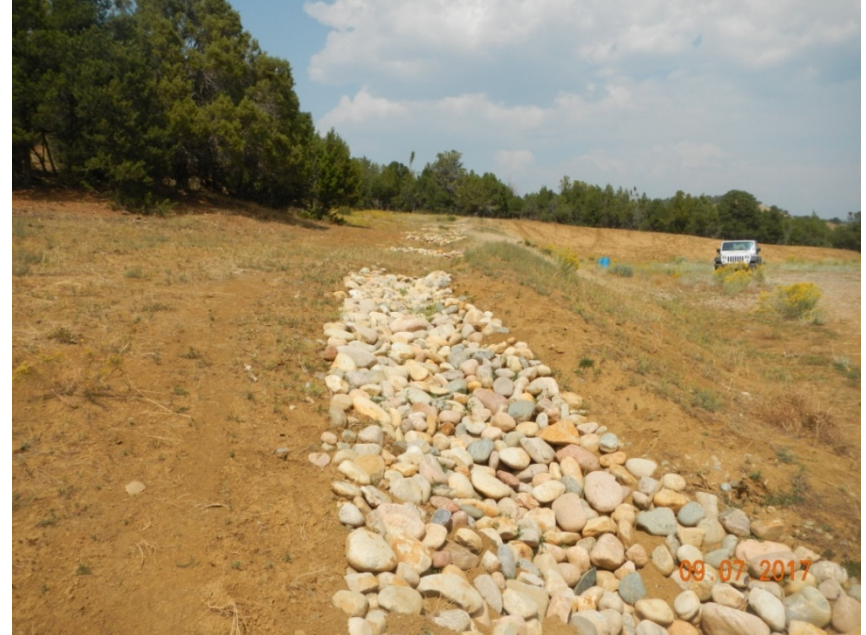
Photo 2: Another view of stormwater controls within the western portion of the project area. Cobble check dams visible in background.
