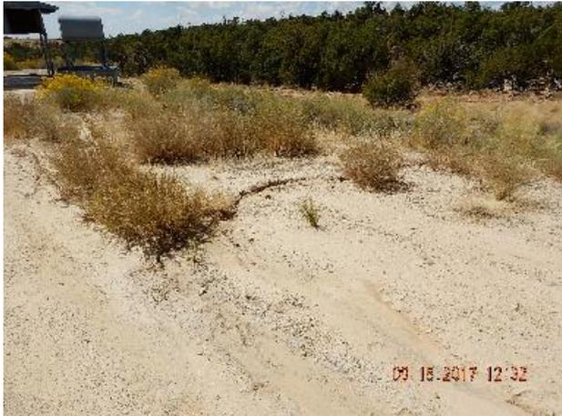
**Photo 9: Stormwater flow coming down access road grade at entrance. Previous inspection.**
