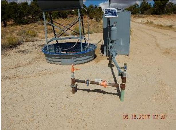
**Photo 5: Line into meter and low point stub up and valve. Previous inspection**
