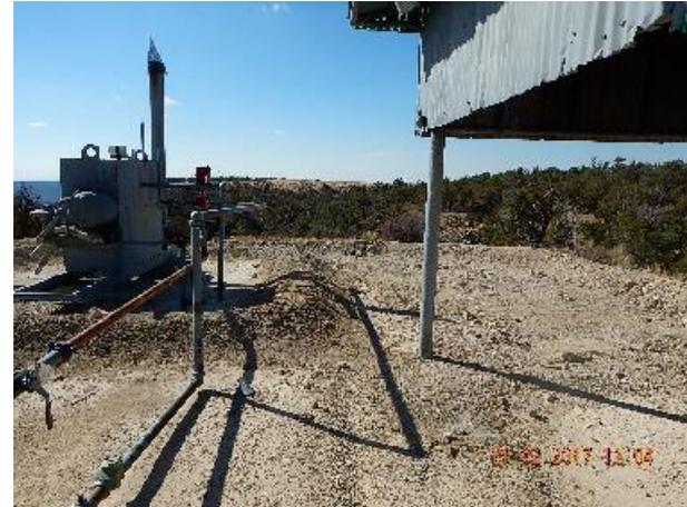
**Photo 14: Repaired surface area and new berm to control stormwater. Follow-up inspection.**
