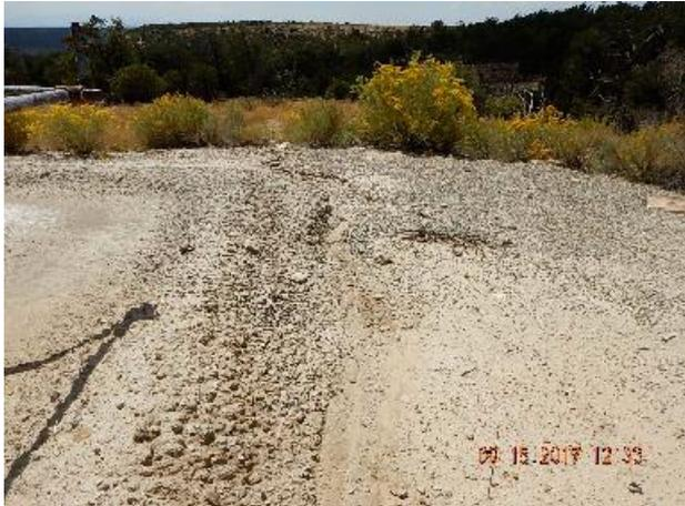
**Photo 13: Erosion channel on SW corner along separator berms. Previous inspection.**
