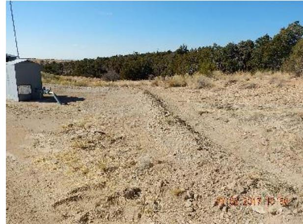
**Photo 10: New diversion berm for stormwater coming off access road. Follow-up inspection.**
