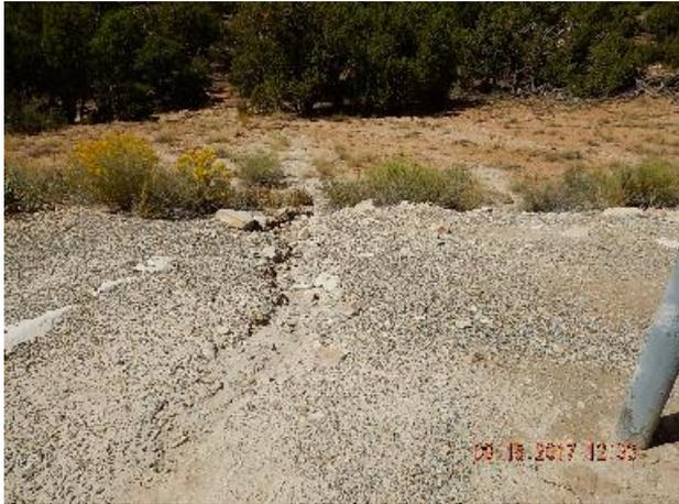
**Photo 11: Erosion channel on SW corner beside carport shelter. Previous inspection.**
