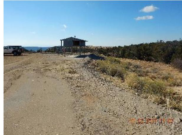
**Photo 12: New berm along perimeter to divert/control stormwater. Follow-up inspection.**
