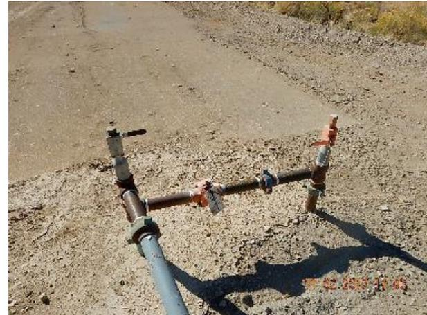
**Photo 6: Line into meter and low point stub up with locked and tagged valve. Follow-up inspection.**
