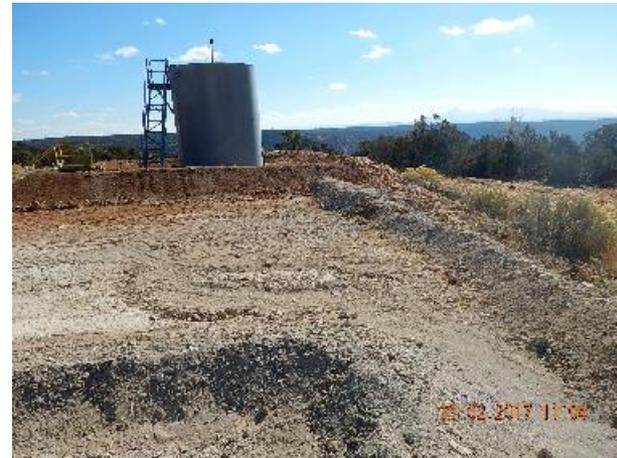
**Photo 8: Repaired surface area and new berm. Follow-up inspection.**
