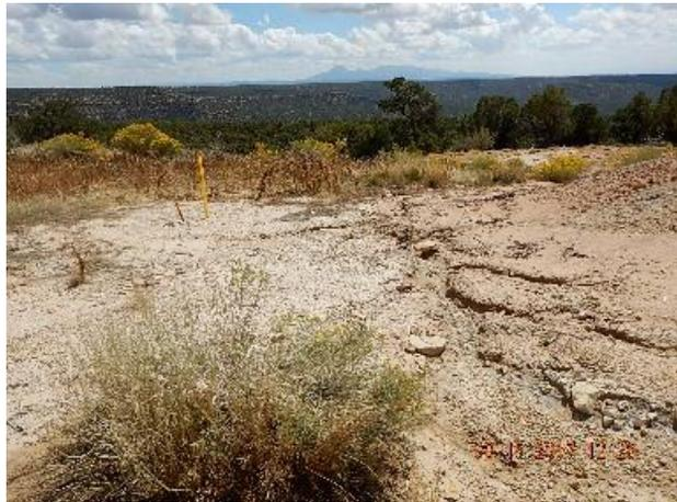
**Photo 7: Stormwater erosion channel off front of production tank berm. Previous inspection.**
