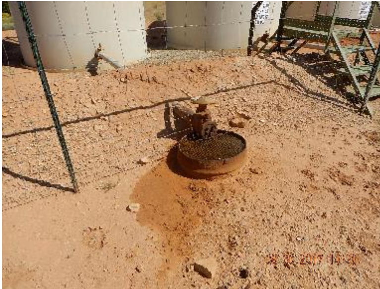
Photo 15: Water tank load out spill prevention full and impacted soil from overflow. Previous inspection.
