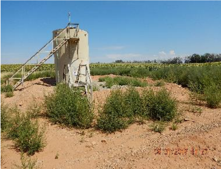
Photo 11: Production tank battery with weeds inside and outside berms. Previous inspection
