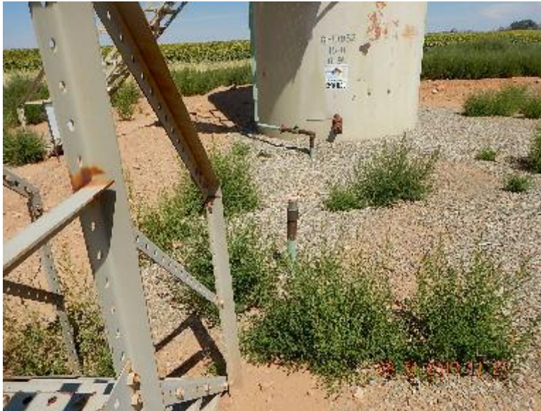
Photo 7: Riser and weeds inside berms of tank battery. Previous inspection.
