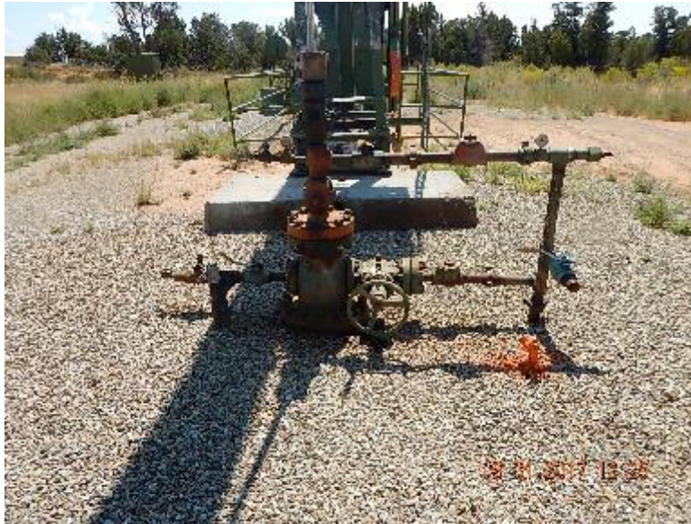
Photo 3: Wellhead and riser. Previous inspection.
