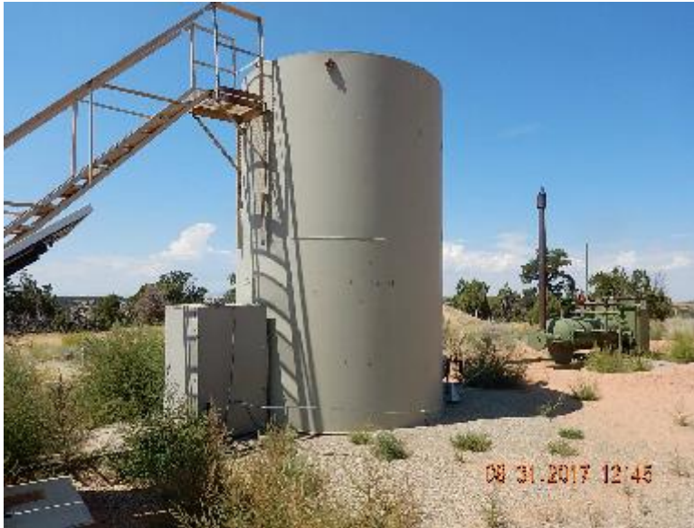
Photo 15: Unlabeled 210 BBL steel tank. Previous inspection.
