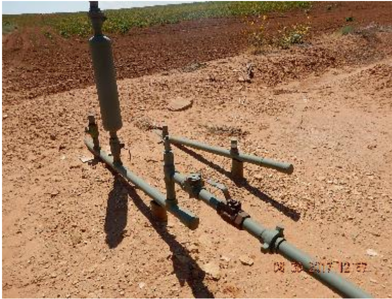
Photo 5: Abandoned flowline on S side of gas meter run building.
