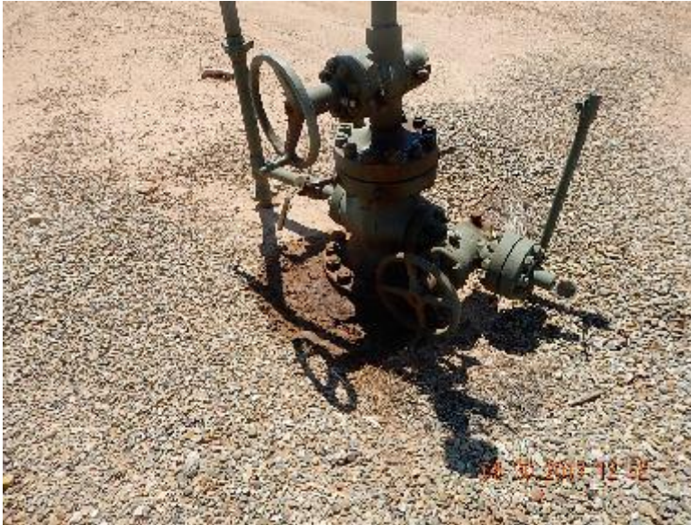
Photo 3: Impacted soil and gravel around base of wellhead.
