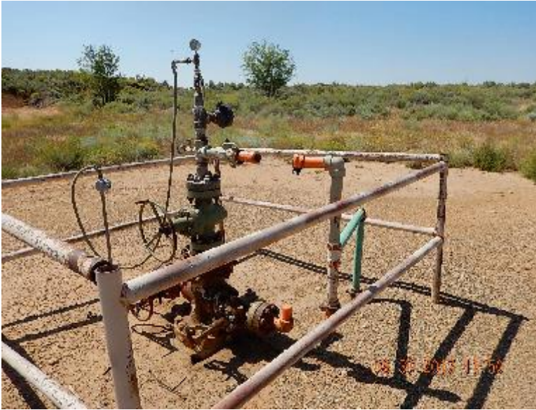
Photo 3: Disconnected wellhead and riser. Previous inspection.
