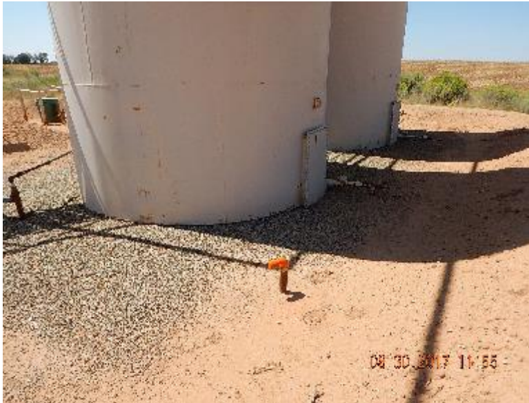
Photo 9: Riser in production tank battery. Previous inspection.
