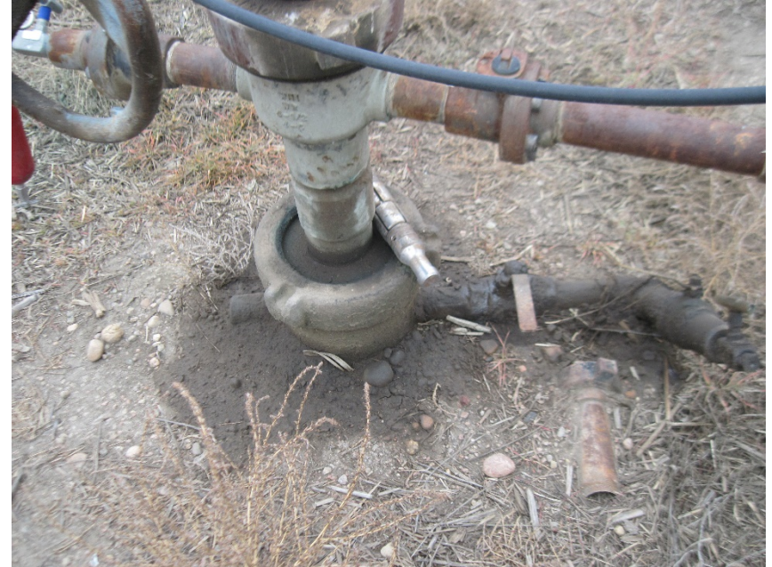
SOILED DIRT AROUND WELLHEAD
