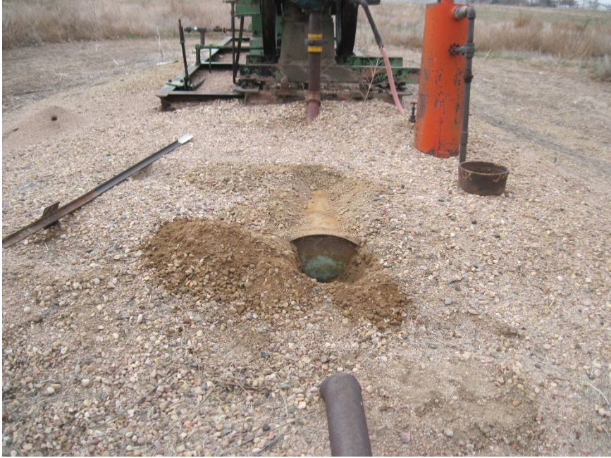
Buried 55 gallon drum need pit permit for this
