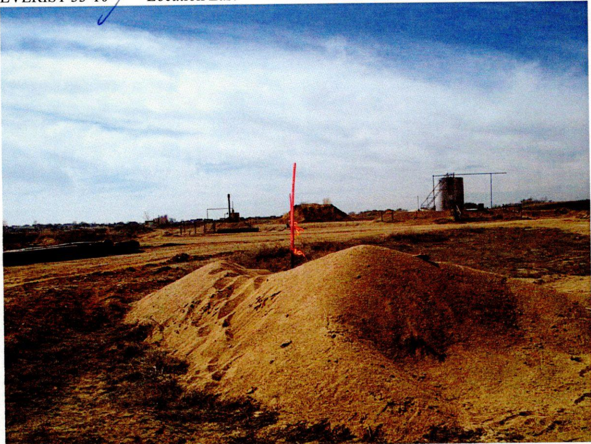
EVERIST 33-10 Access South
