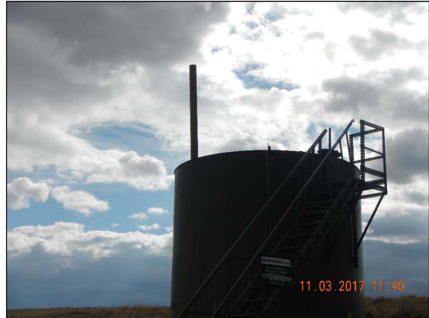
Photo 2. No wildlife protection on tank exhaust.
