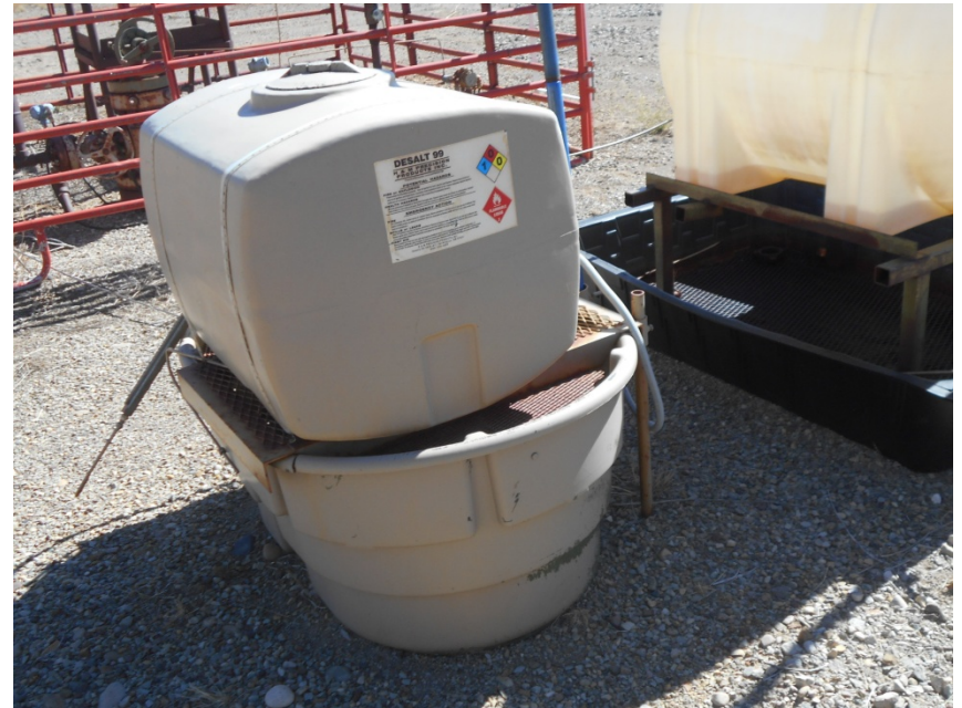
Chemical drums with secondary containment. Picture taken 10/23/2017
