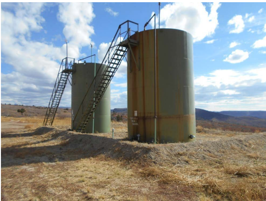
Tank berms before corrective action. Picture taken 11/3/2016
