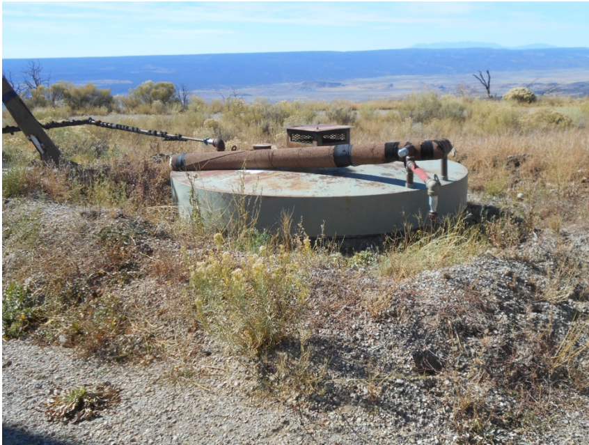
Reboiler water line disconnected from tank.
