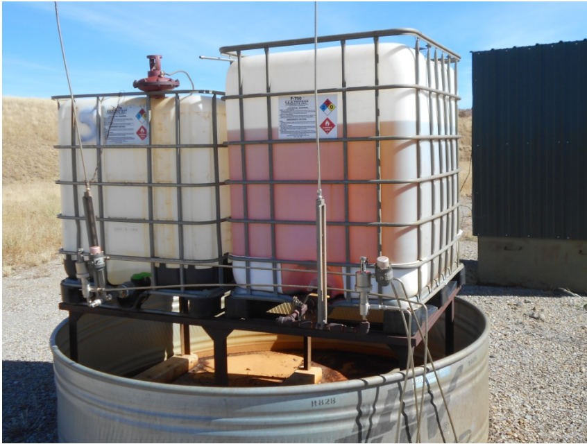
Chemical drums with secondary containment. Picture taken 10/23/2017
