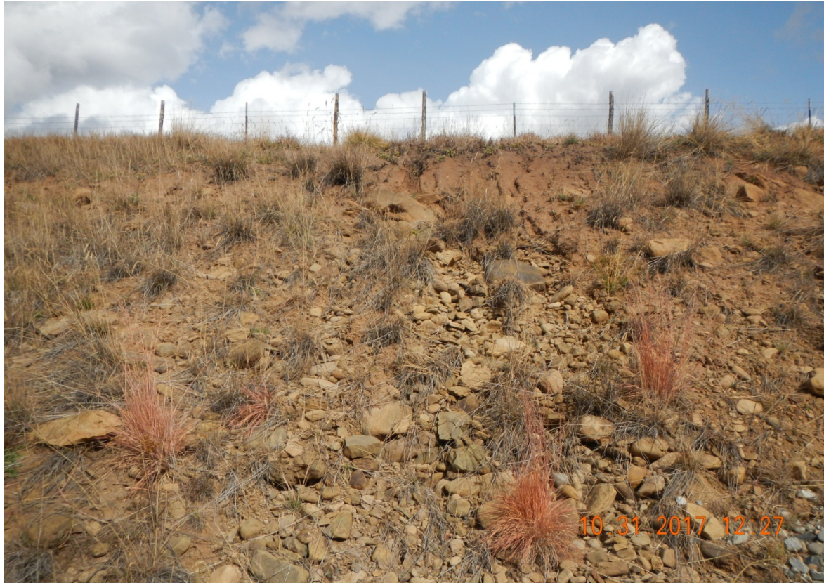
Ope Photo 3 Erosion on Cut Slope of location
