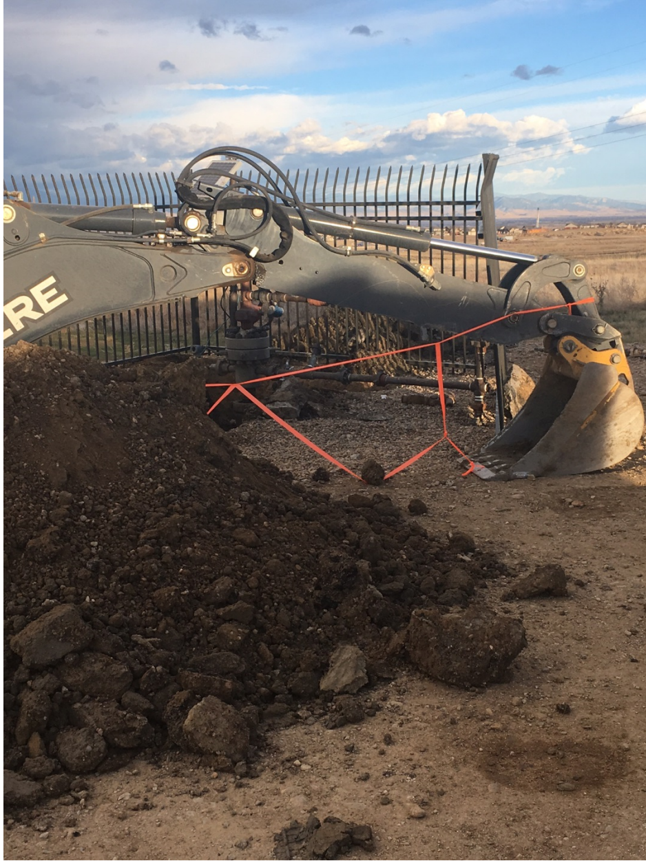
Removal around wellhead
