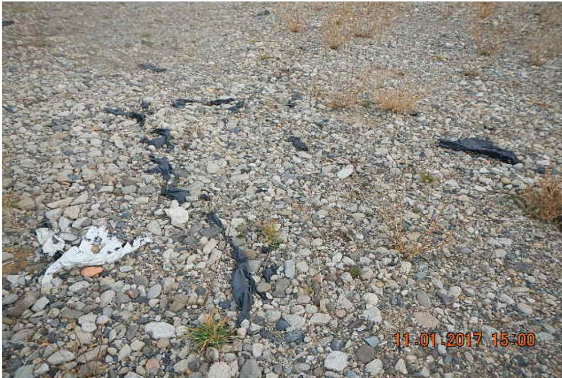
**Photo 5 Debris incorporated with fill**
