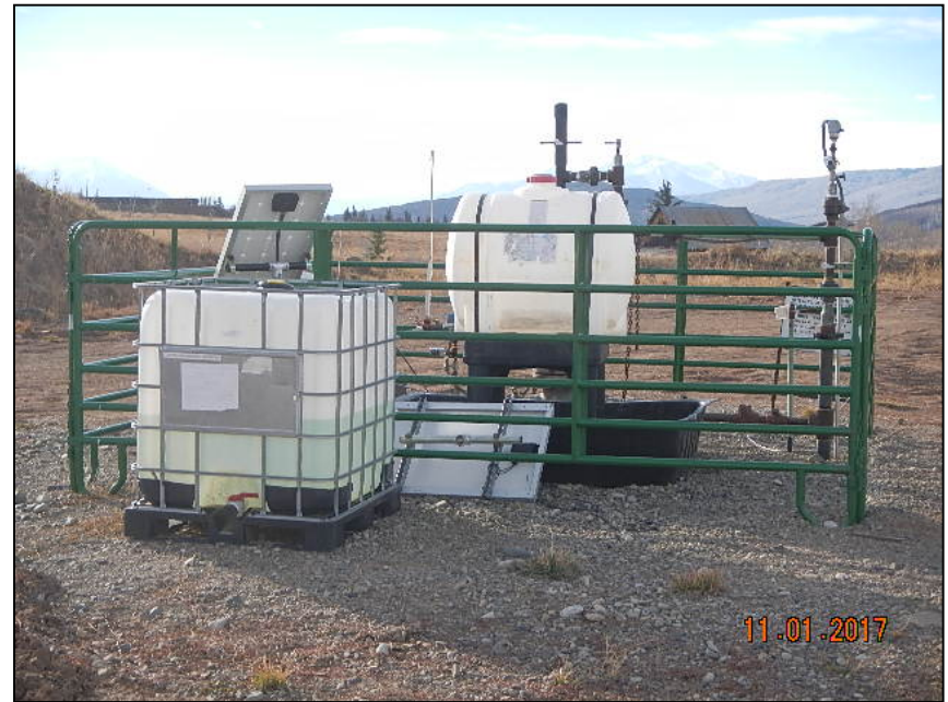
Photo 2. Stored chemical container.
