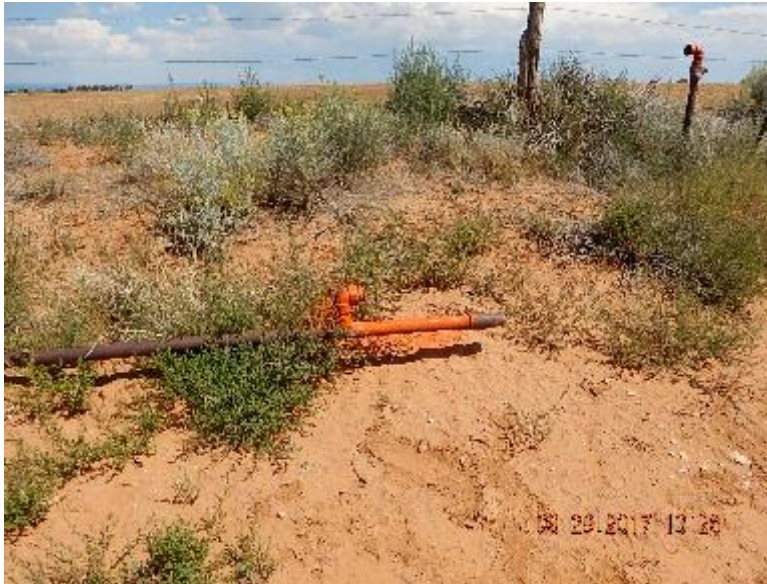
Photo 9: Open ended line and riser behind gas meter run house. Previous inspection.
