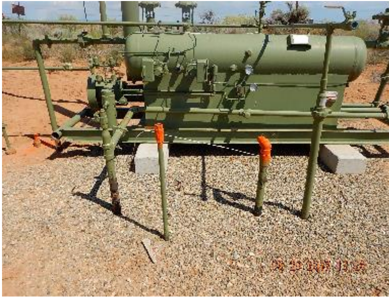
Photo 13. : Risers on W side of separator. Previous inspection.
