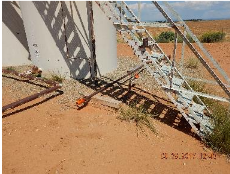
Photo 15. : Risers and patches of grass inside production tank battery. Previous inspection.
