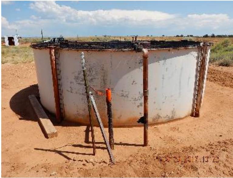
Photo 5: Riser at produced water open top tank. Previous inspection.
