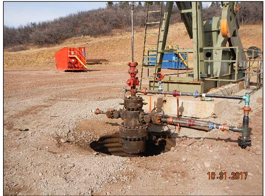
Photo 8. No sign at wellhead. Staining on wellhead and in cellar.
