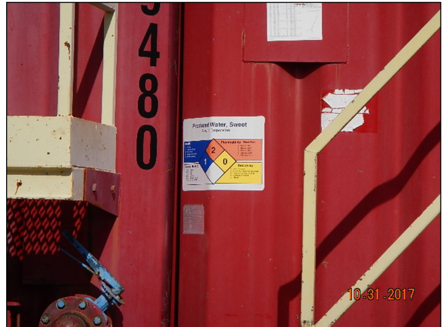
Photo 2. Incorrect signage on unused tanks.
