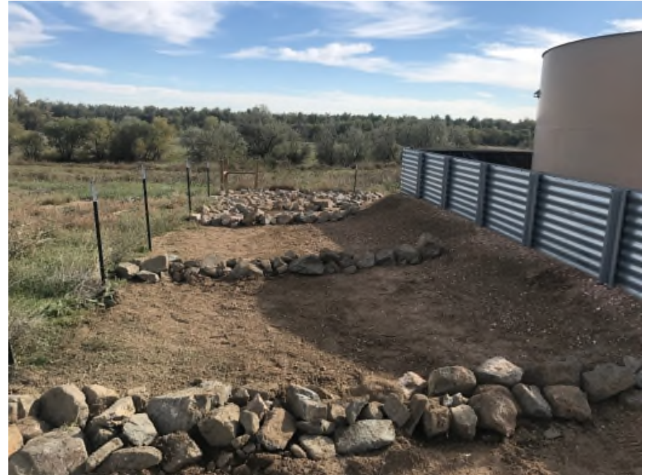
Photo NBL1. Discharged sediment was recovered. The rills were repaired and new BMPs (check dams) were installed. Noble also installed rip rap in the corner of the pad to prevent future sediment loss.
