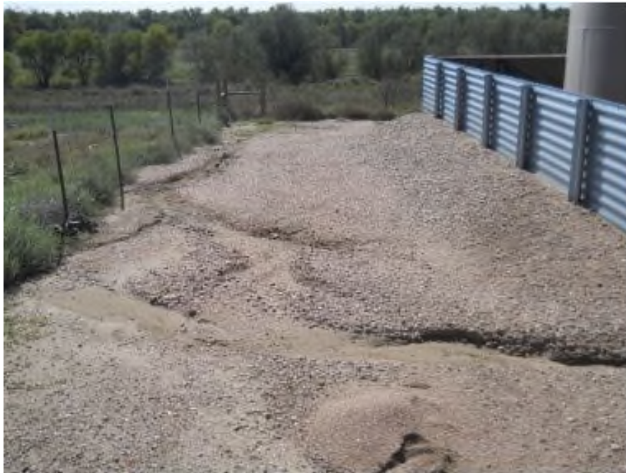
Photo 5: Location washing out from northeast edge of tank battery and running along the east side of tank battery, discharging sediment off of location
