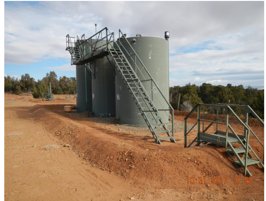
Produced water ASTs.
