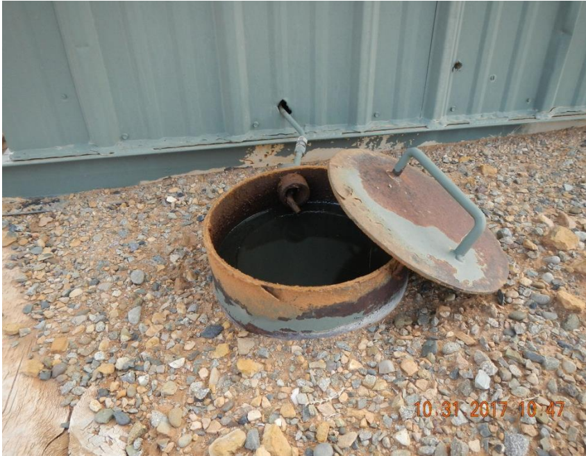
Drain line sump for meter house.
