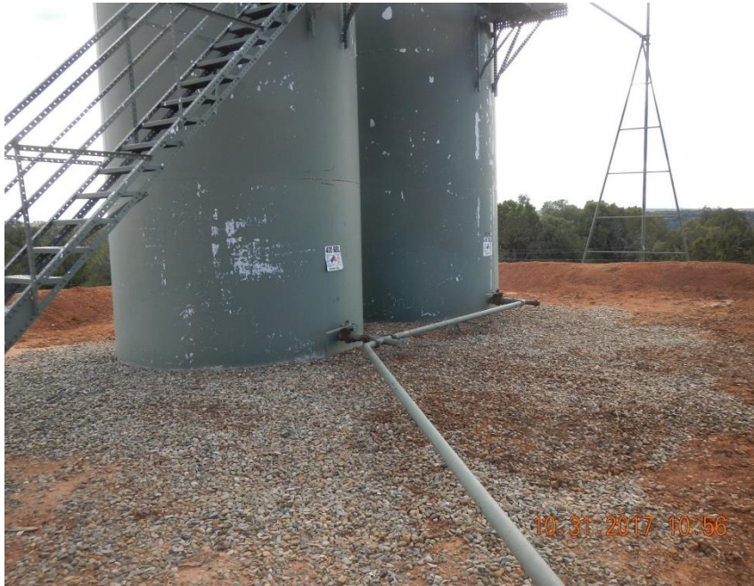
Secondary containment area for crude oil tanks. Samples were reportedly collected from in front of tanks.
