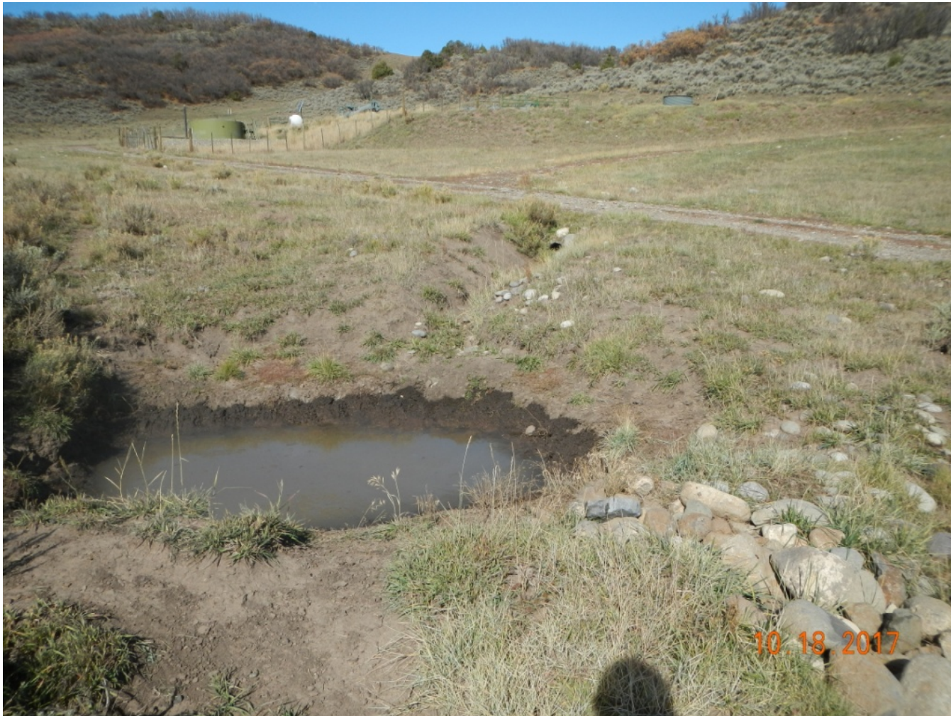
Photo 5. View of another silt trap at the southwestern edge of the project area, appears to be functioning.
