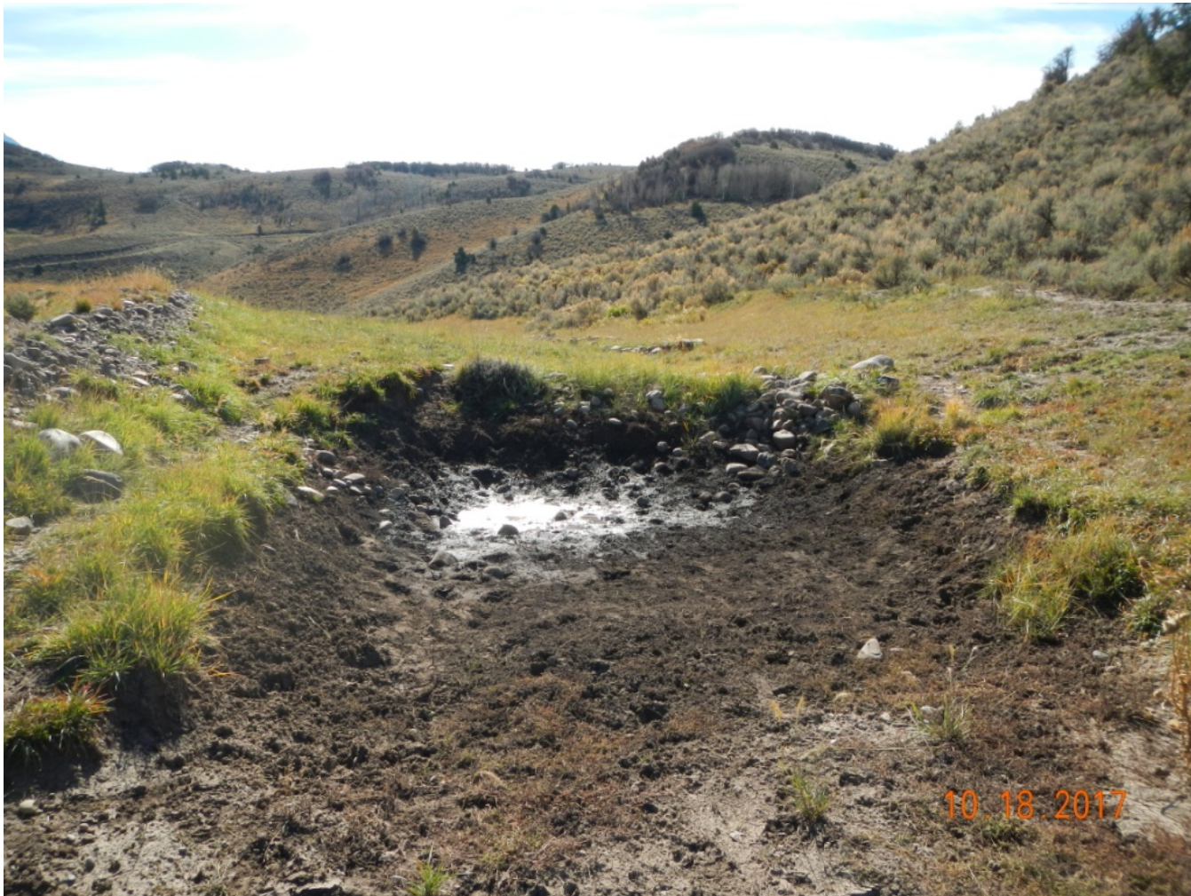
Photo 4. View of silt trap in the southern portion of the project area that appears to recently have been maintained.
