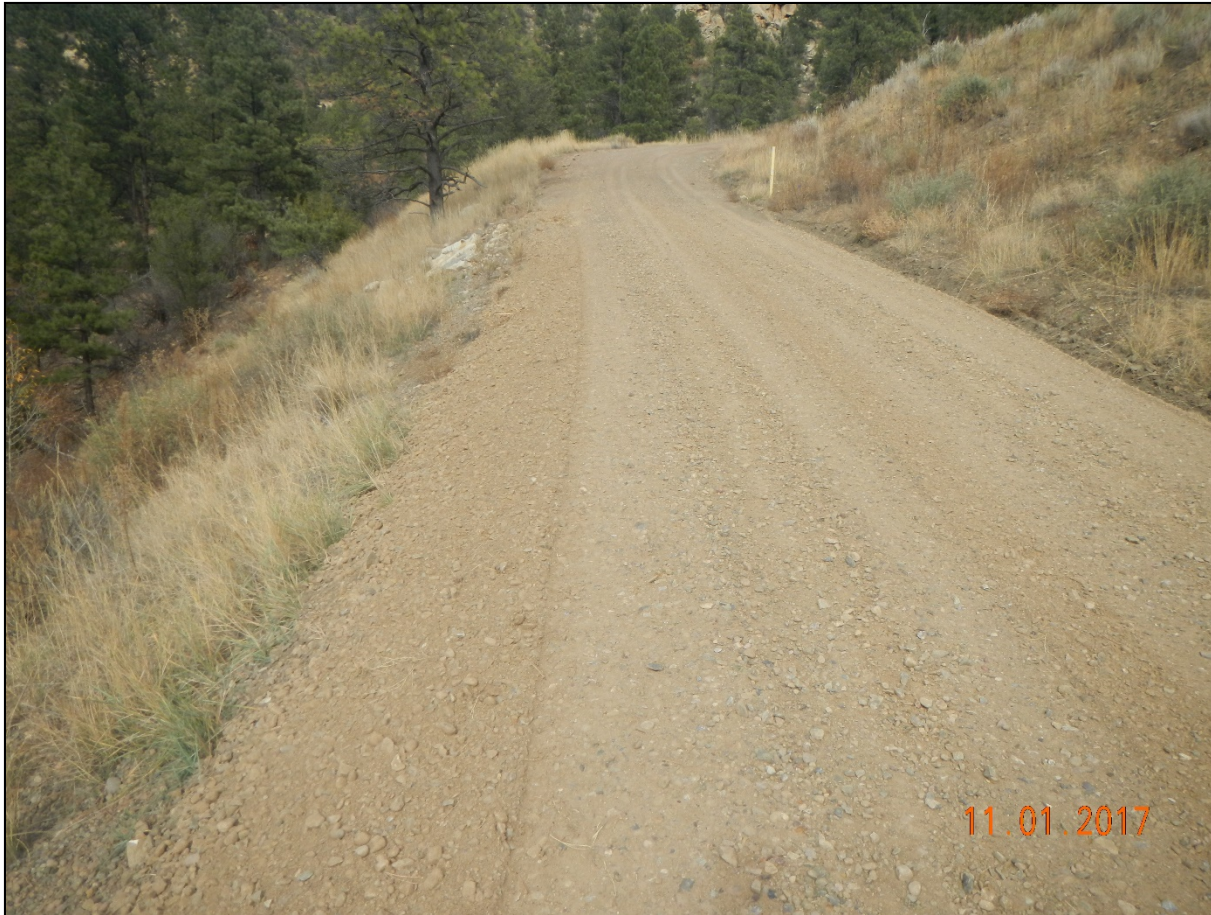
Photo 6. Facing north along the access road. Gravel material has been applied to areas along the road.
