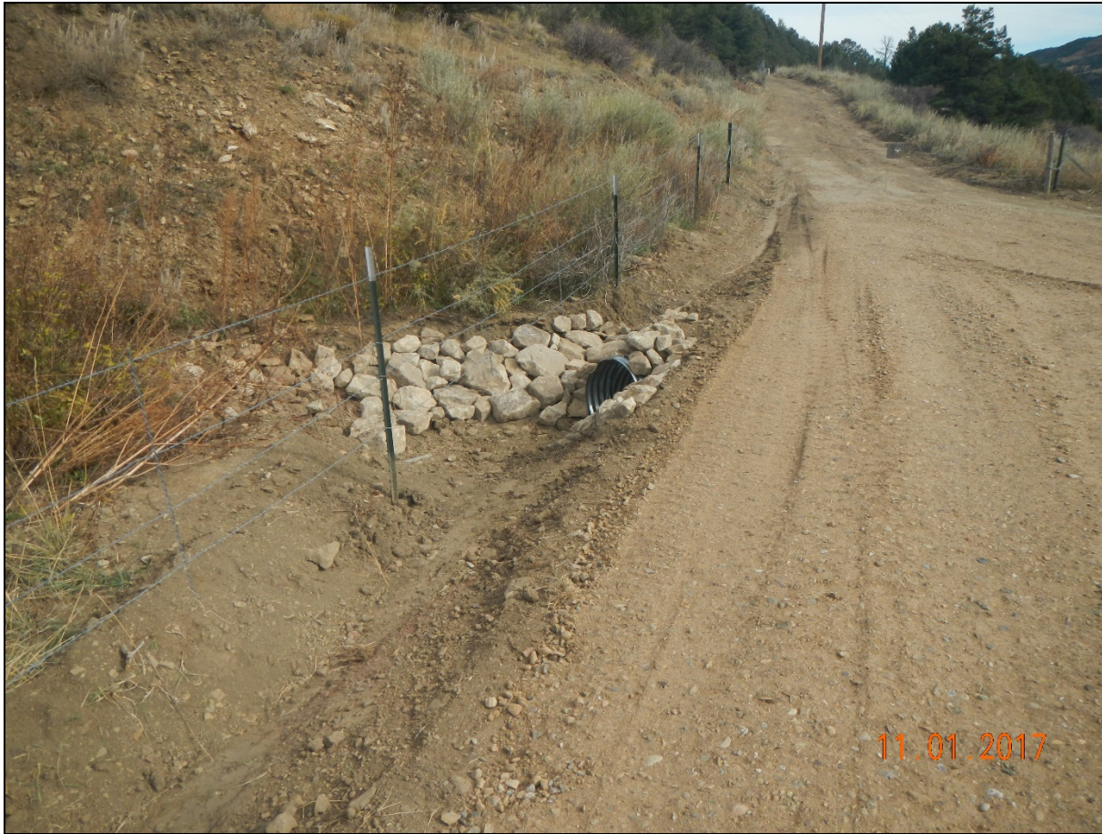
Photo 2. A culvert was installed to direct stormwater away from the access road and highway.
