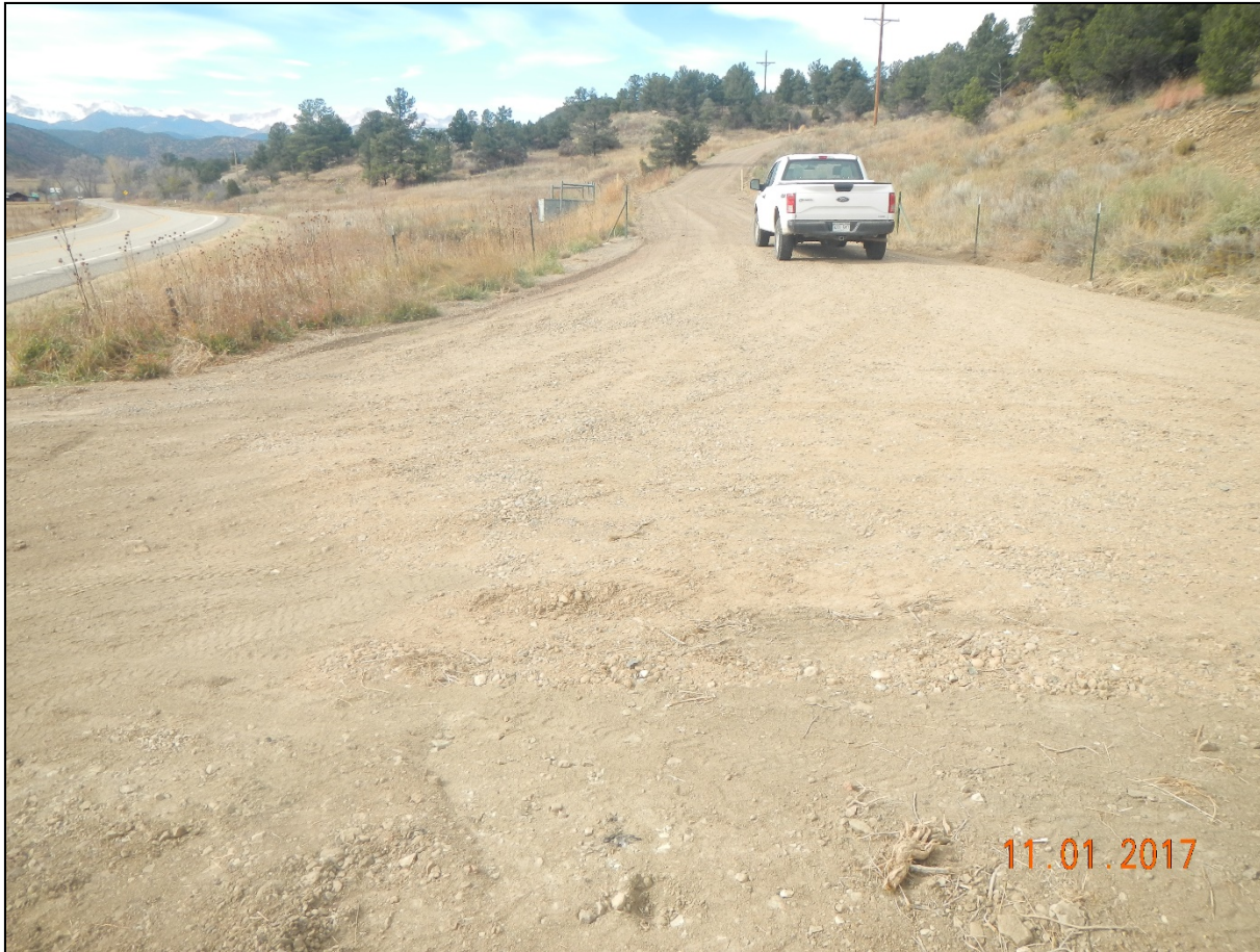
Photo 1. Facing northwest at the beginning of the access road standing near Hwy 12. Gravel has been applied and compacted to the surface to prevent vehicle tracking..
