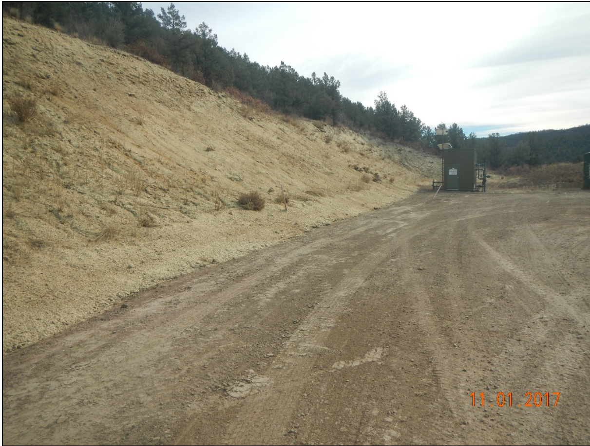
Photo 7. Facing southeast at the location toward the cut slope. The cut slope is temporarily stabilized with hydro-mulch.
