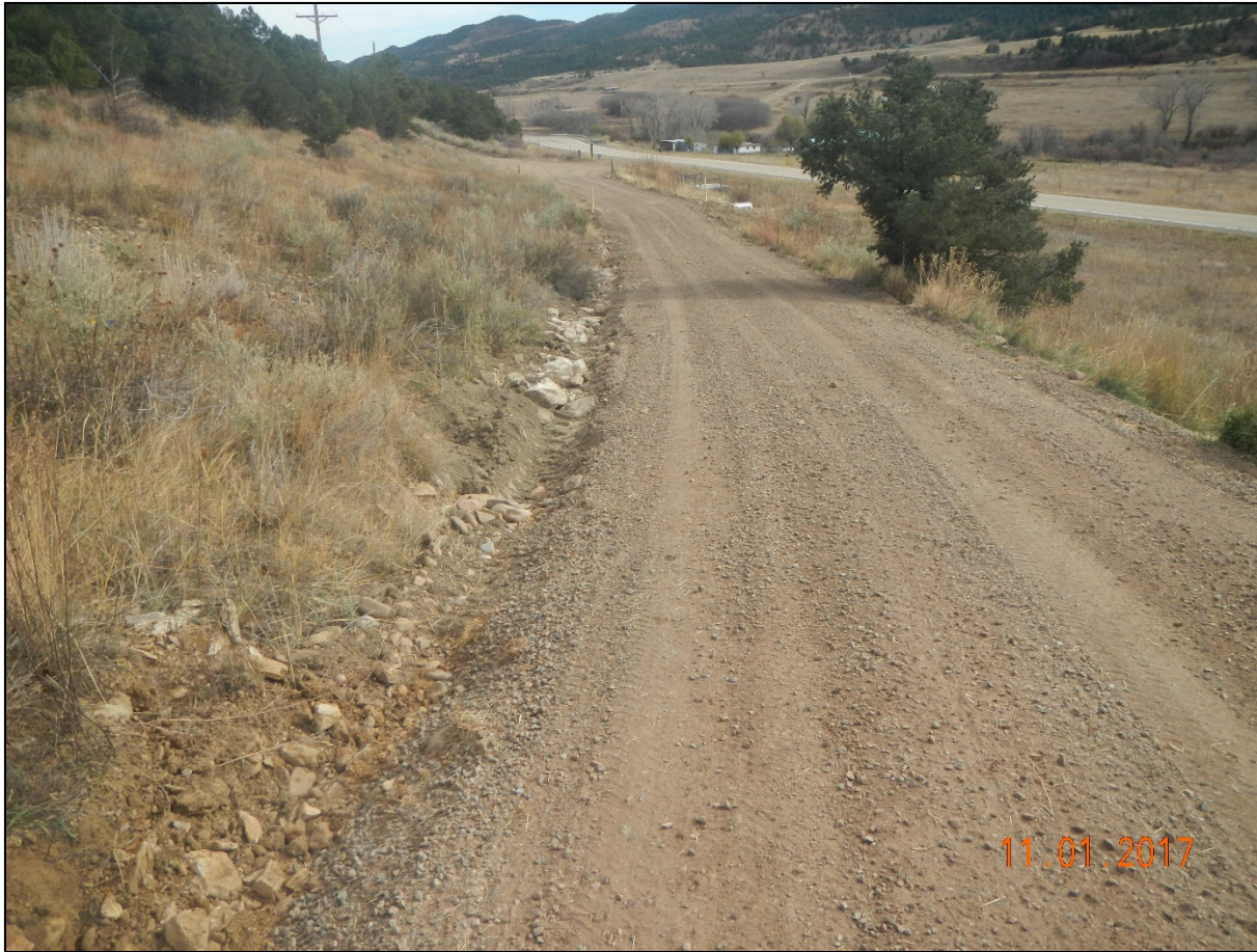
Photo 5. The side of the access road has been filled in where it was eroded. Some rock rip/rap has been placed to prevent erosion.
