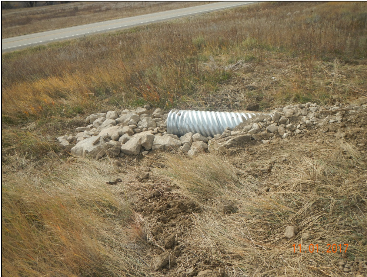
Photo 4. The culvert was installed with rock rip/rap outlet protection.
