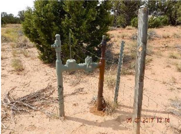
**Photo 7: Impacted soil at riser by location entrance previous inspection.**
