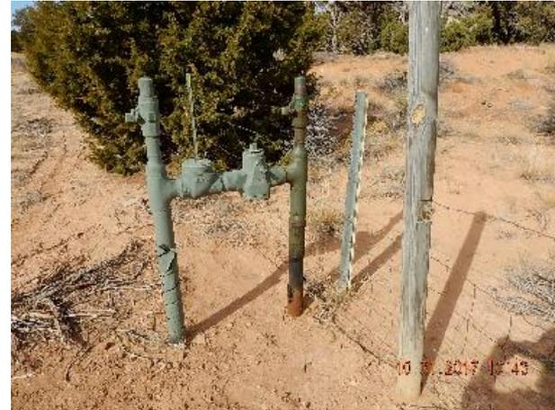
**Photo 8: Cleaned up impacted soil at riser by location entrance. Valve and bull plug tightened. Follow-up inspection.**
