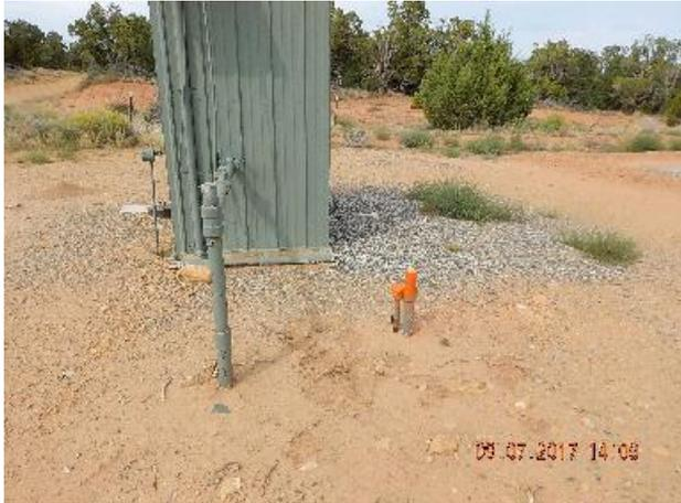
**Photo 11: Unused risers at gas meter shed previous inspection.**
