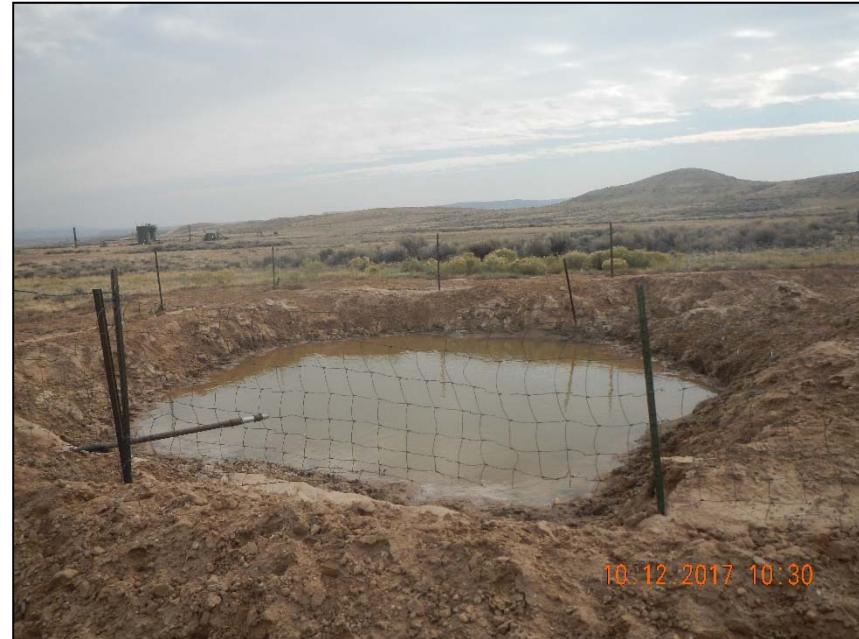
Photo 2. View of pit facing northeast.
