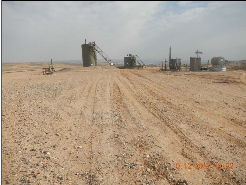
Photo 1. View of location facing southwest.
